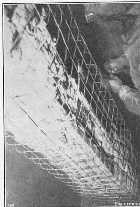
FIG. 5. PLACING WIRE MESH ROUND PILE.
