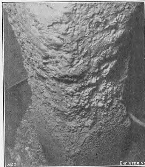
FIG. 2. PILE READY FOR TREATMENT.
