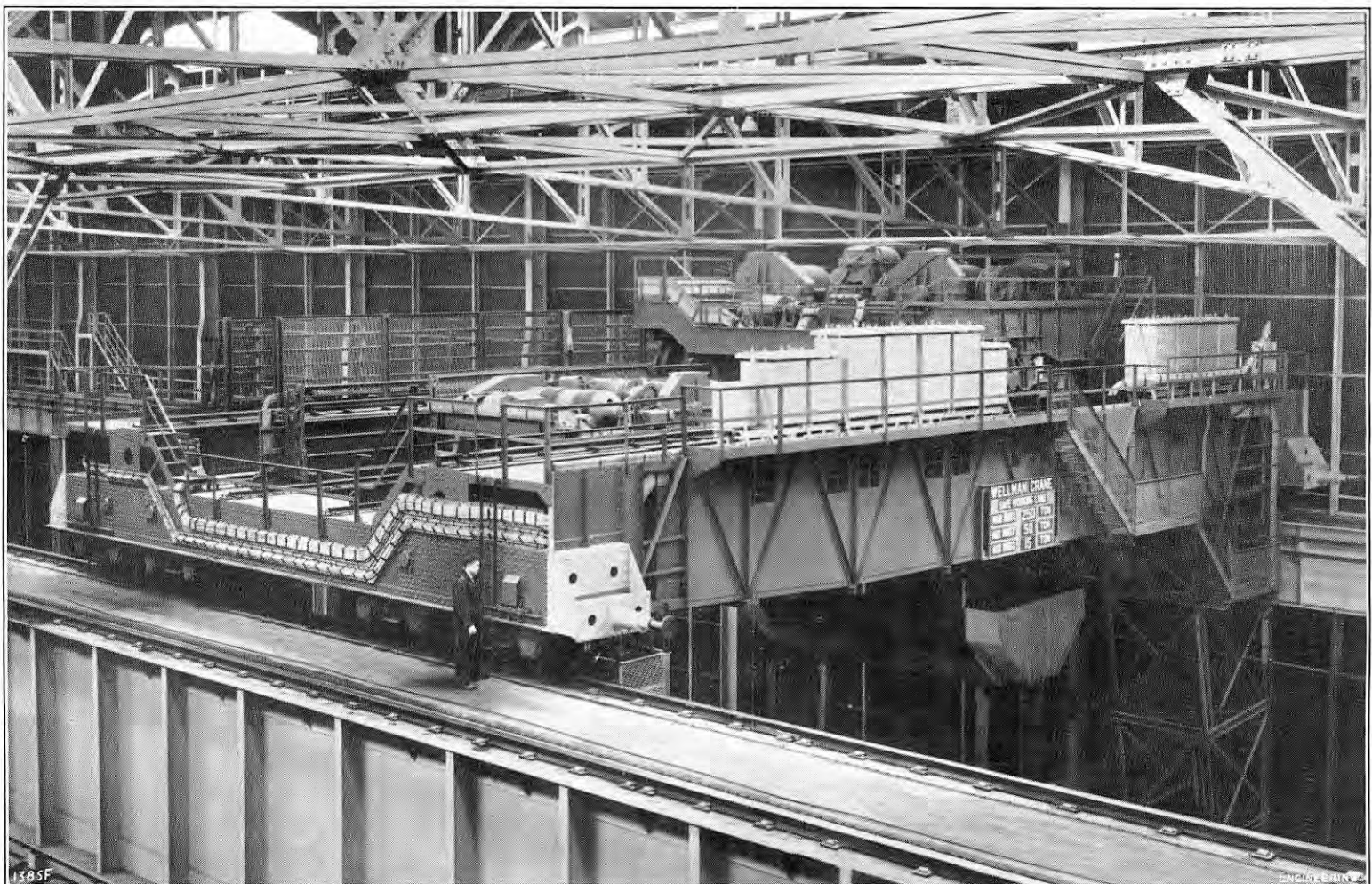
FIG. 6. 250-TON CRANE, SHOWING MAIN AND AUXILIARY TROLLEYS.
