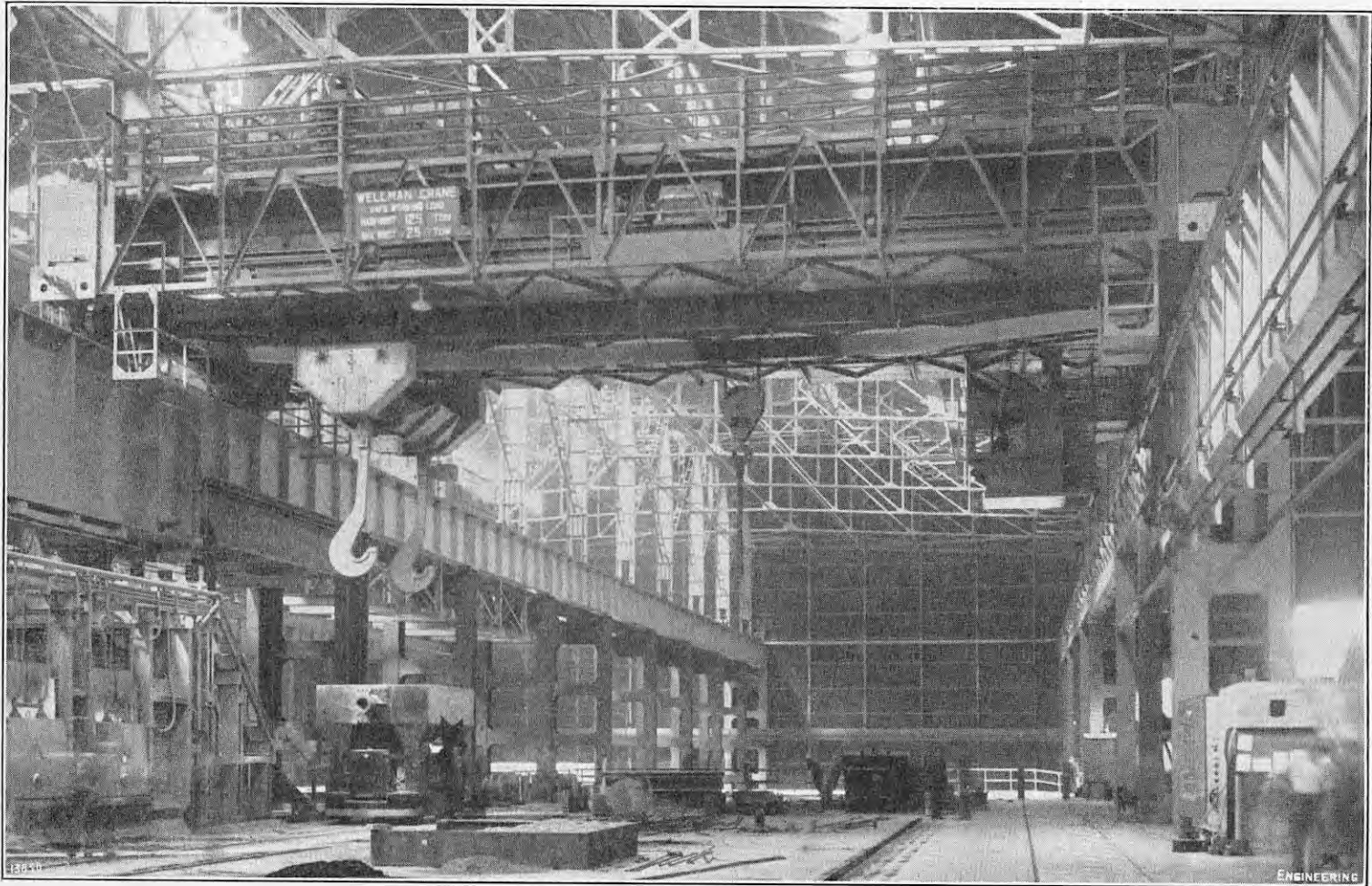
FIG. 3. 125-TON HOT-METAL LADLE CRANE.
