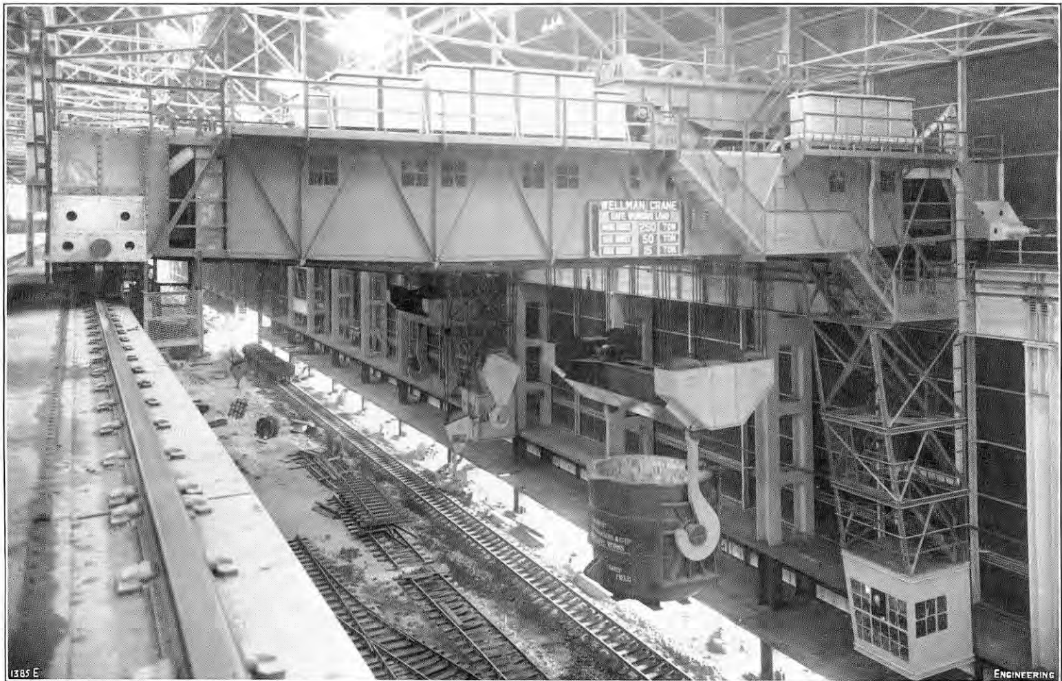
FIG. 5. TWO 250-TON LADLE CRANES IN STEELWORKS.
