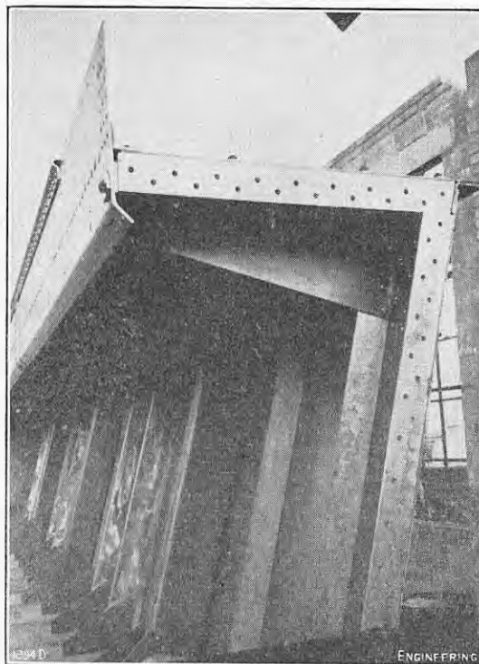
FIG. 4. COAMING AND JOINING ANGLE.
