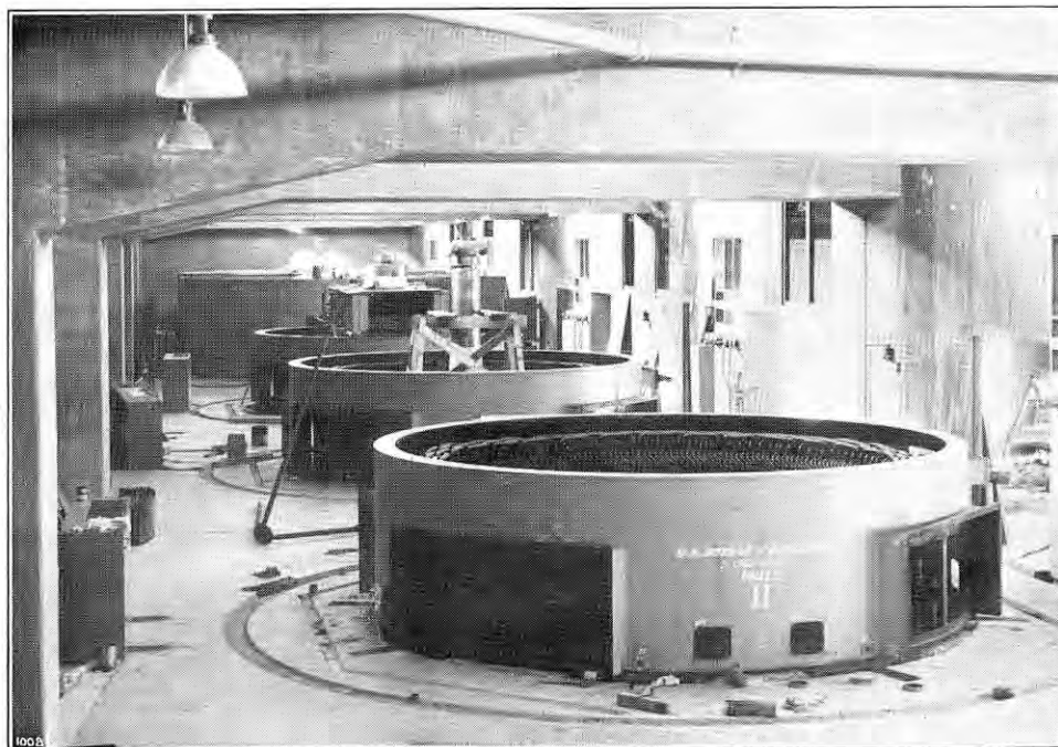
FIG. 16. FIRST THREE MOTORS DURING ERECTION.
