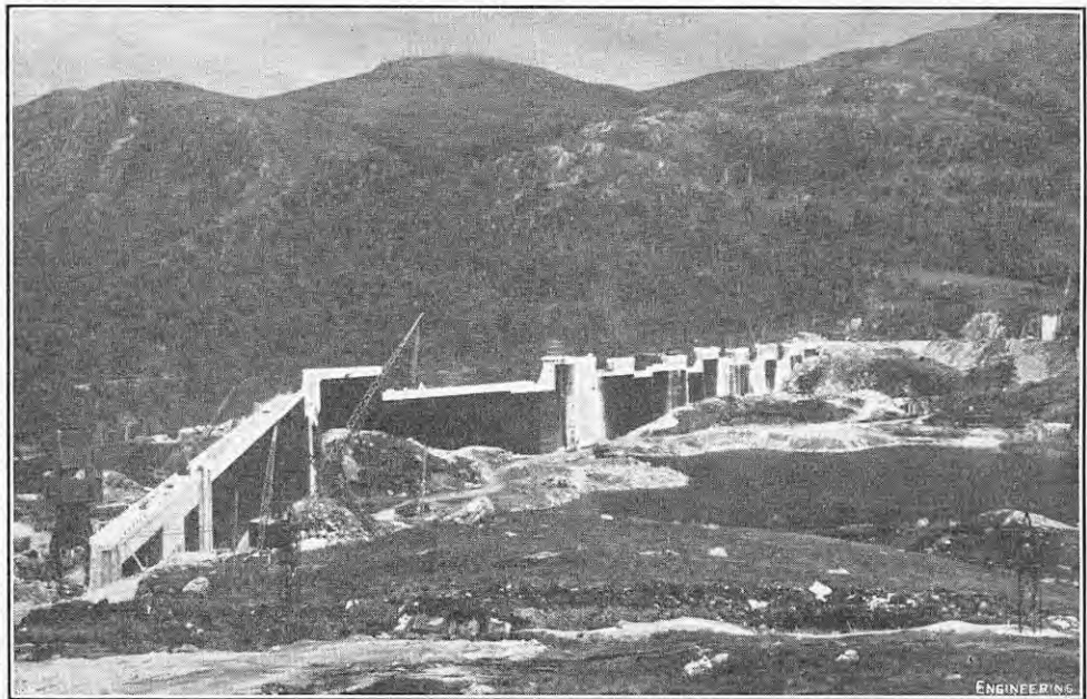
FIG. 3. MULLARDOCH DAM UNDER CONSTRUCTION.
