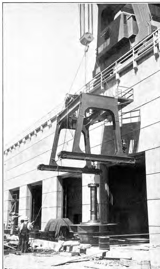
FIG. 13. JACKING FRAME HANDLING PUMP IMPELLER.
