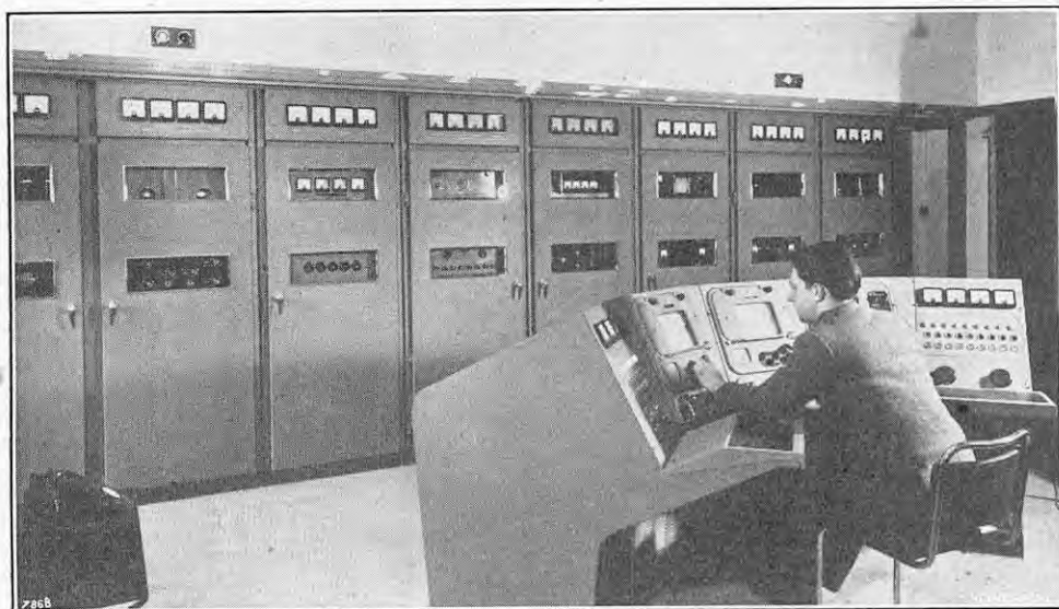
FIG. 2. CONTROL DESK AND MEDIUM-POWER TRANSMITTERS.
