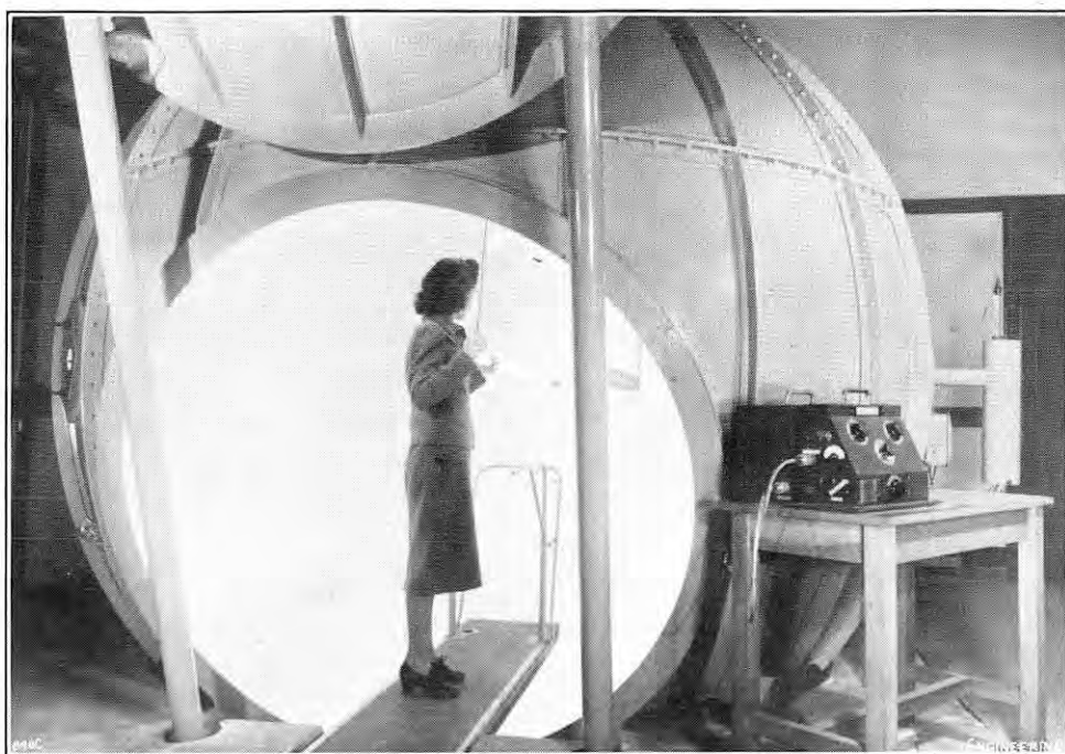
FIG. 32. 12-FT. SPHERICAL INTEGRATING PHOTOMETER; GENERAL ELECTRIC CO., LTD.
