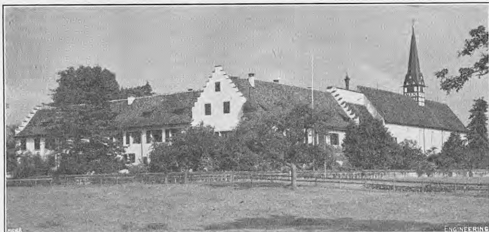
FIG. 1. PARADISE ESTATE BUILDINGS.
