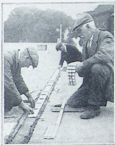
Mr. R. F. Brown (right) superintending the laying of his patented white line at Clacton-on-Sea. The line is made up of cubes of hard clay with centre cubes of glass.
