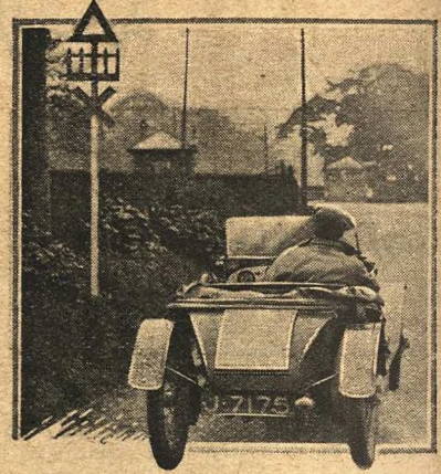
A unique triple warning erected on the Blaydon road near Newcastle. The top denotes dangerous corner, the centre sign a level crossing, and the bottom cross roads.
