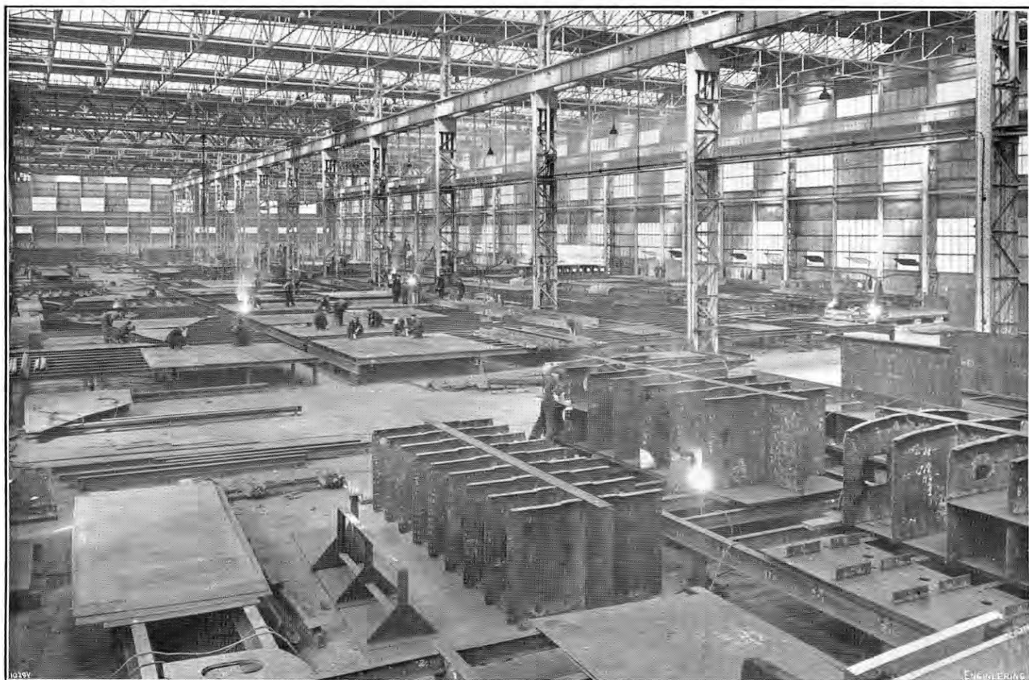
FIG. 23. WELDING SHOP AT QUEEN'S ISLAND.
