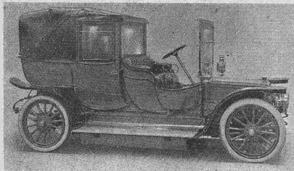
Fig. 2.—The most noticeable feature is the front extension, providing shelter for the front seat. Detachable and hinged aluminium extension pieces connect the front screen to that behind the driver, forming grooved ways for the flexible roof-piece. A stiffening cross-member is provided to these coupling pieces.
