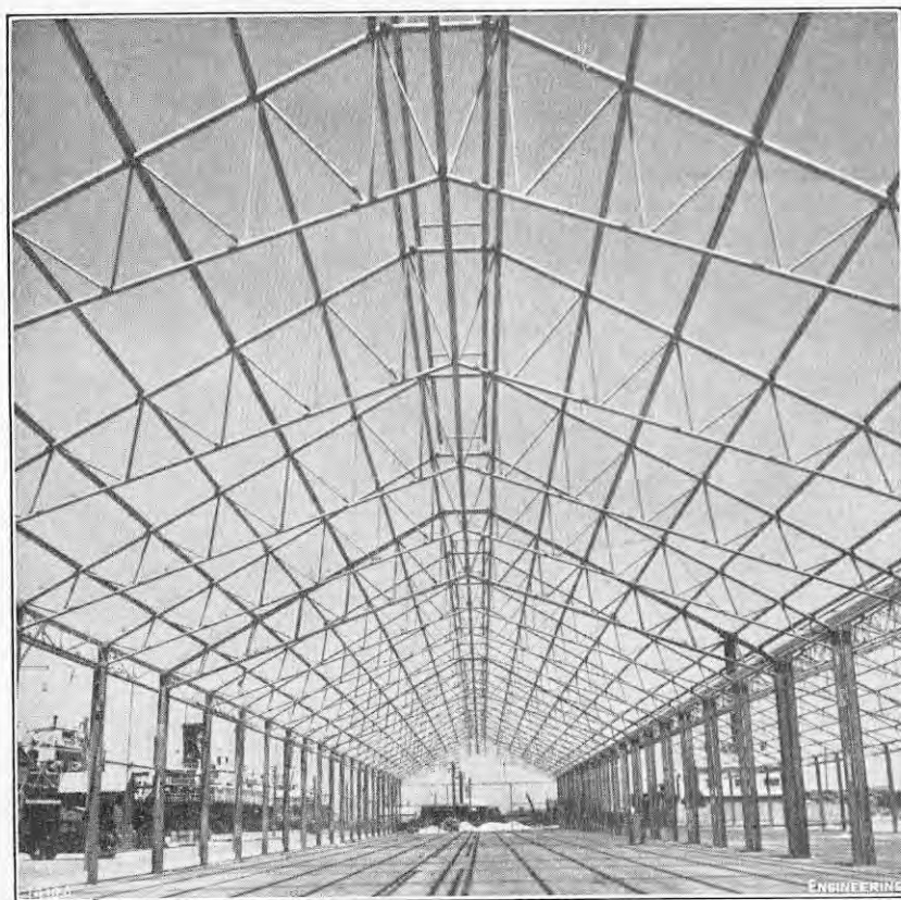
FIG. 1. "ARCON" STORAGE BUILDING UNDER CONSTRUCTION.
