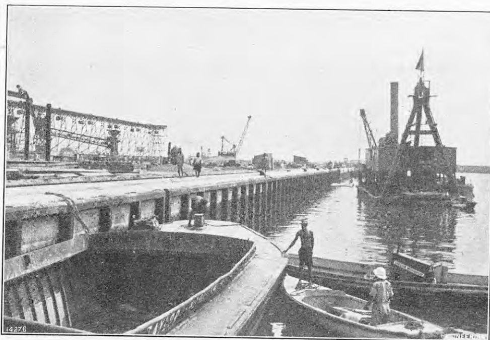
FIG. 3. TIMBER FENDERING TO WHARF EXTENSION.
