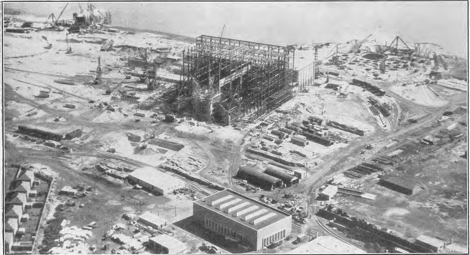
FIG. 1. GENERAL VIEW OF SITE.
