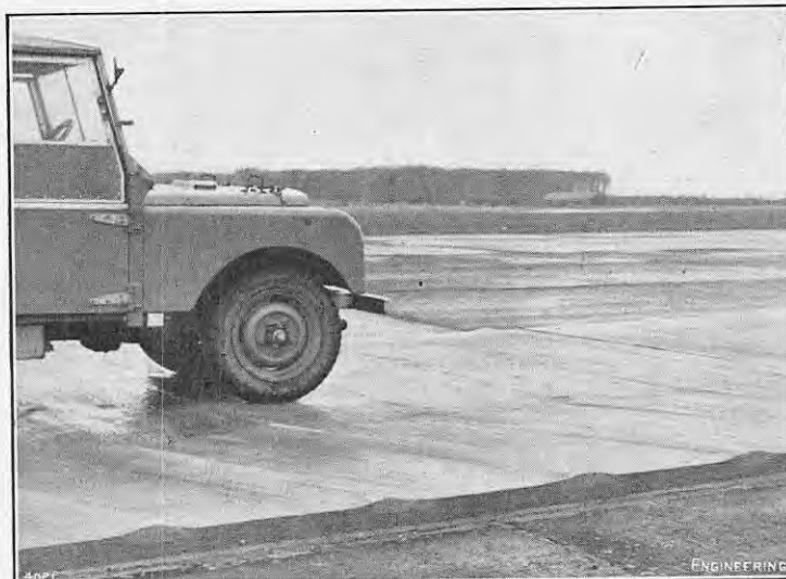
FIG. 3. CORRUGATED ROAD SURFACE.
