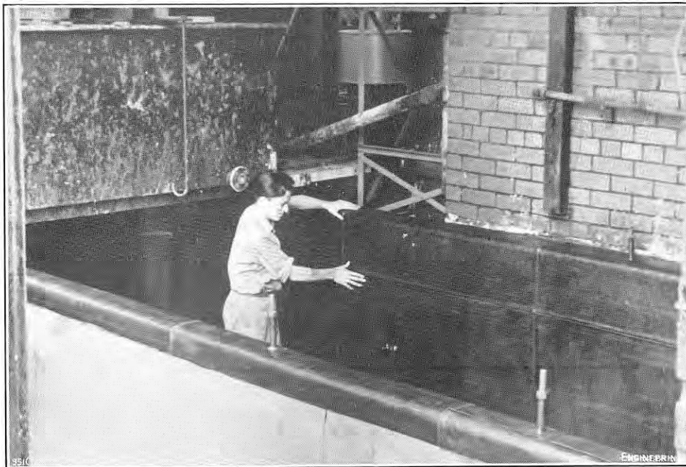
FIG. 3. CONCRETE TANK LINED WITH P.V.C.
