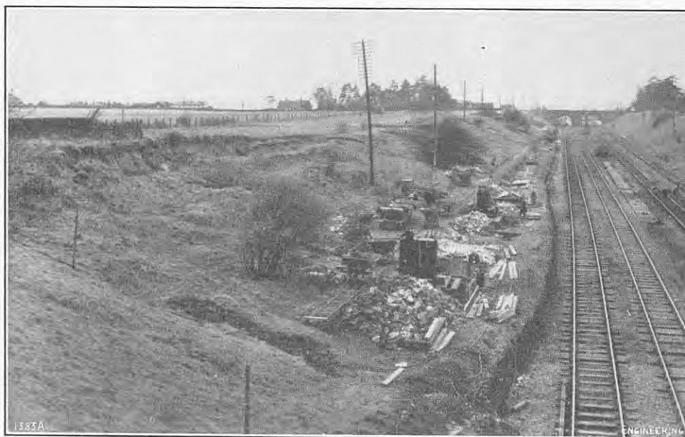
FIG. 1. THE SLIP AT TWYFORD.
