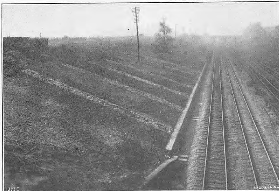
FIG. 3. RESTORED EMBANKMENT AT TWYFORD.
