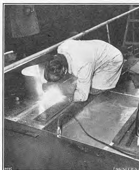
FIG. 3. DOWN-HAND WELDING OF ROOF PLATING.
