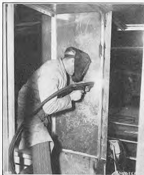
FIG. 2. TACK WELDING PLATE TO STANCHIONS.
