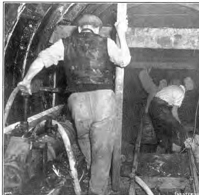
FIG. 14. EXCAVATION OF COOLING-WATER TUNNEL.
