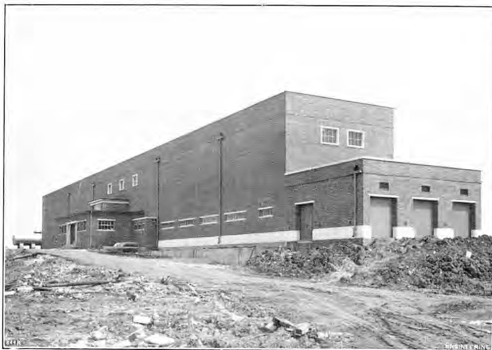
FIG. 11. MAIN PUMP HOUSE.
