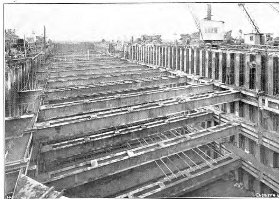
FIG. 17. EXCAVATION FOR PUMP HOUSE.
