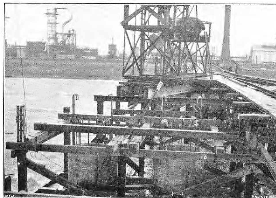
FIG. 23. NEW JETTY UNDER CONSTRUCTION.
