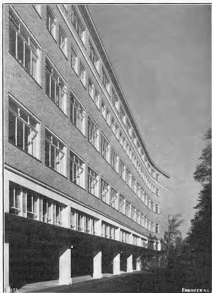
[FIG. 1. EAST ELEVATION FROM SOUTH.]
