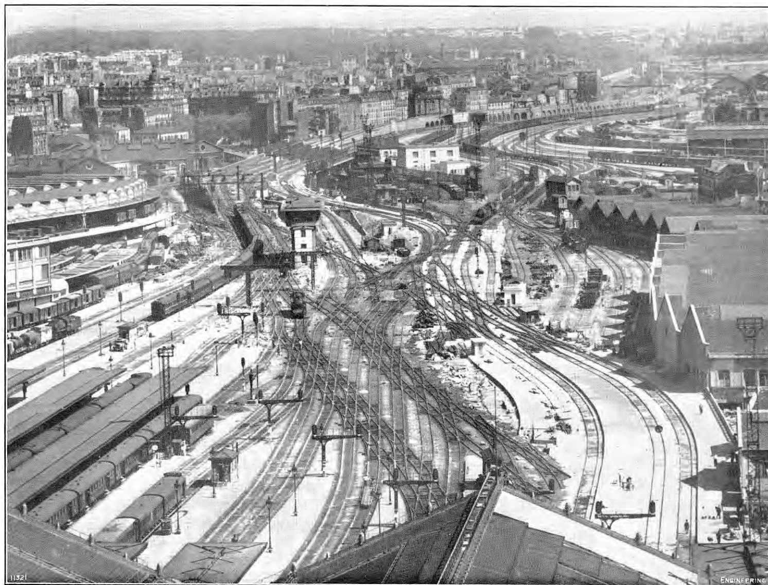
FIG. 9. RECONSTRUCTED APPROACH TO GARE DE LYON, PARIS.
