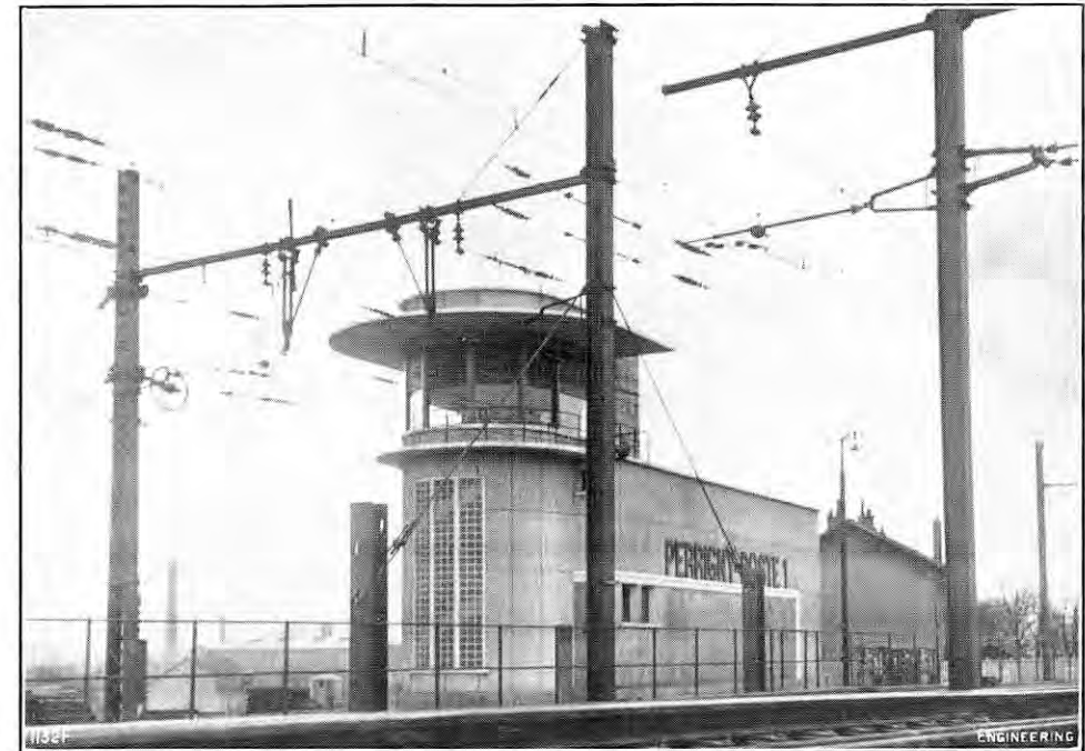
FIG. 6. PERRIGNY SIGNAL BOX.
