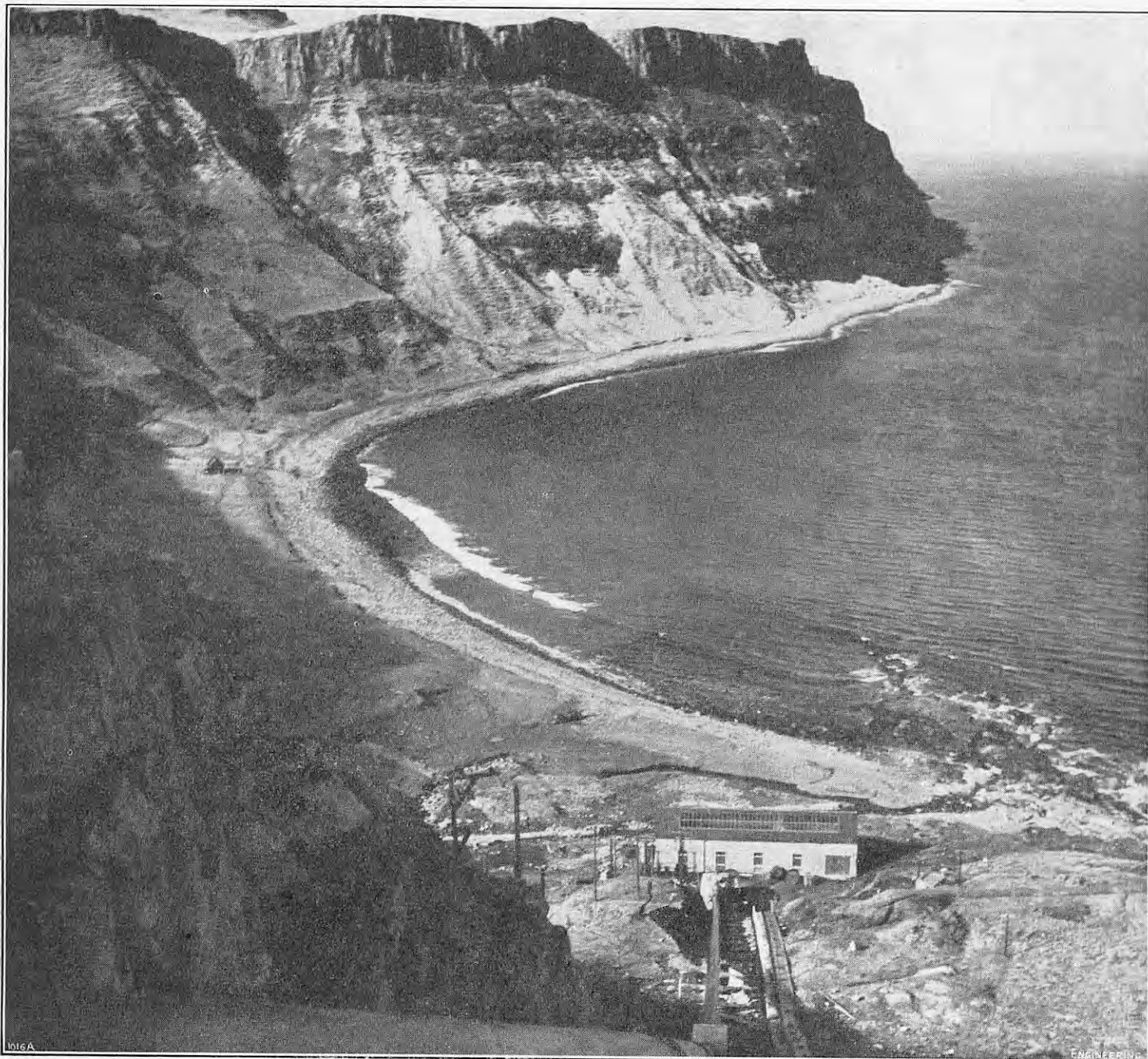
FIG. 1. STORR LOCHS POWER STATION, ISLAND OF SKYE.
