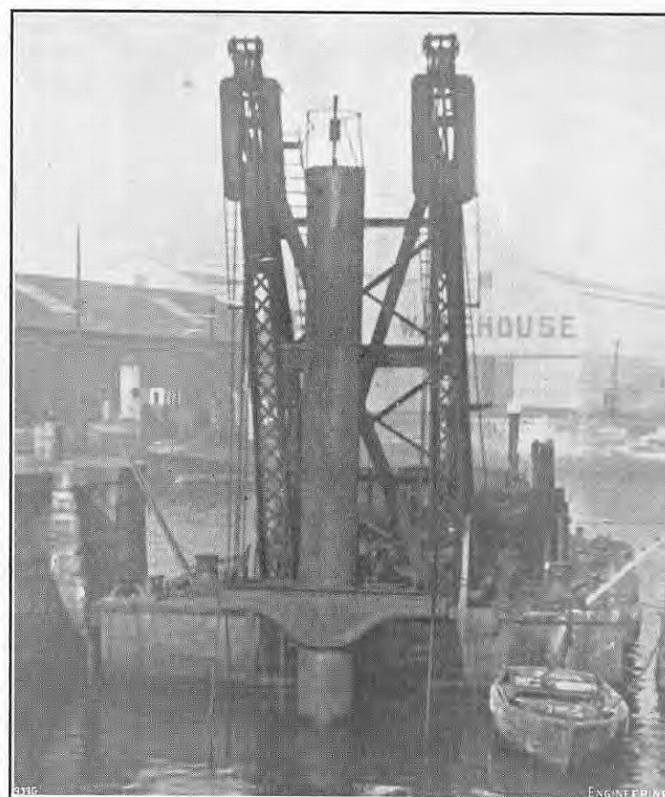
FIG. 7. SUPERSTRUCTURE OF DIVING BELL.
