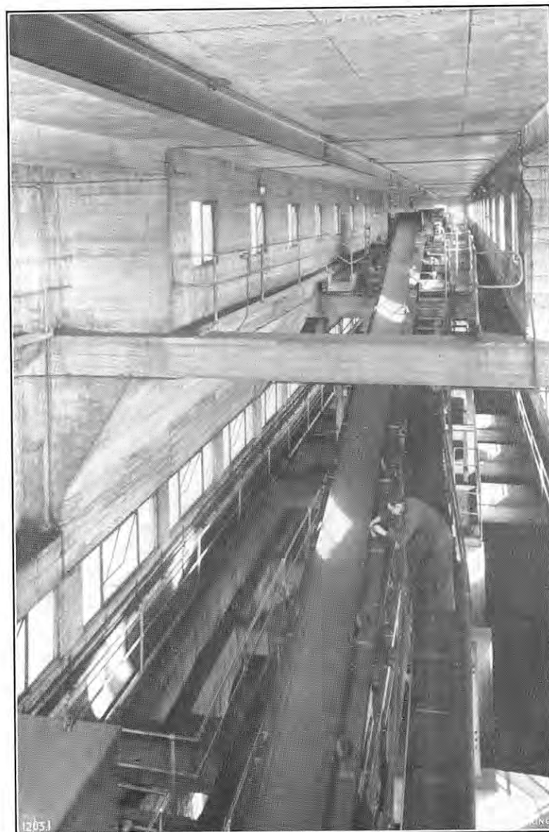
FIG. 10. INTERIOR OF COKE STORAGE BUNKERS.
