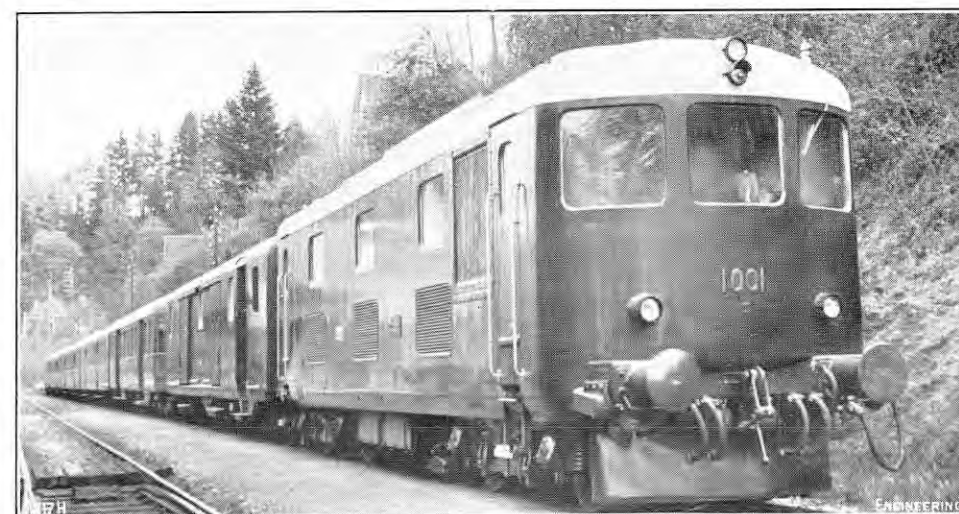
FIG. 8. 1,200-H.P. DIESEL-ELECTRIC LOCOMOTIVE; SWISS FEDERAL RAILWAYS.
