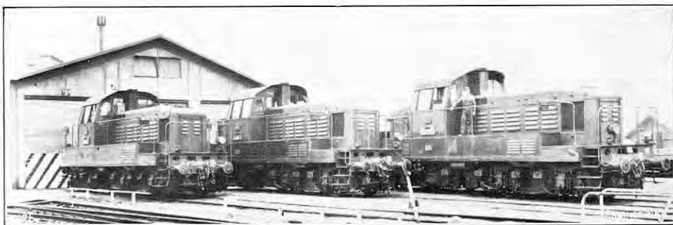
FIG. 5. 735-H.P. DIESEL-ELECTRIC SHUNTING LOCOMOTIVE; FRENCH RAILWAYS.
