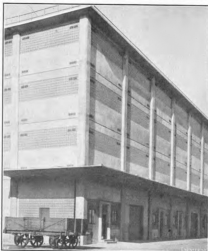
FIG. 6. HARBOUR BOARD'S NEW WAREHOUSE.
