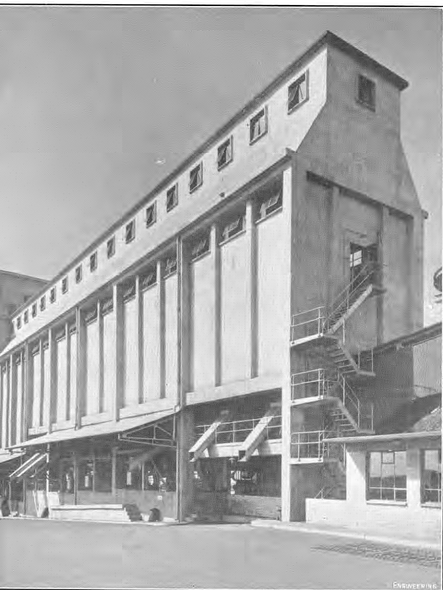
FIG. 11. COKE STORAGE BUNKERS.
