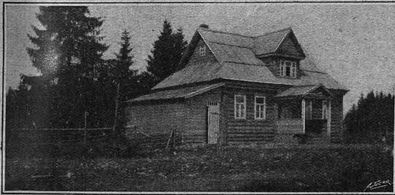
An unfinished house, totally without furniture, in which the writer of the accompanying article found his most comfortable accommodation in 800 miles. Although he had to sleep on bare boards he was consoled by these at least being clean.
