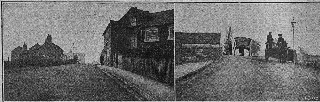
On Saturday last the road from Shrewsbury to Chester, via Hadnall, was closed to all vehicular traffic, probably for some months, as the two narrow bridges which span the Shropshire Union Canal are to be replaced by wider ones. The map above indicates the position of the bridges and also the routes which may be taken either on leaving or entering Shrewsbury to avoid the blocked road. The photographs show, on the left the Factory Bridge and on the right the Comet Bridge which are to be replaced.
