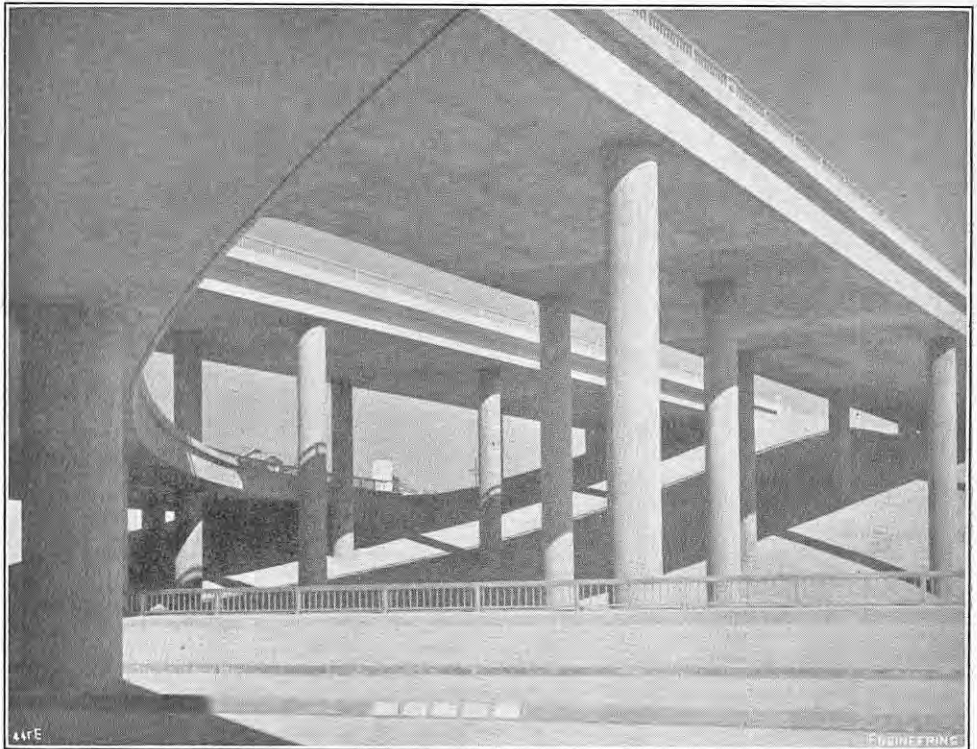
FIG. 5. TOP LEVEL AND TURNING RAMP.
