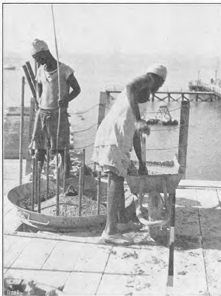
FIG. 7. FILLING CONCRETE PILE.
