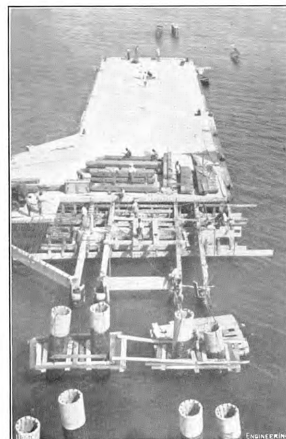
FIG. 18. CONSTRUCTION OF DECK.
