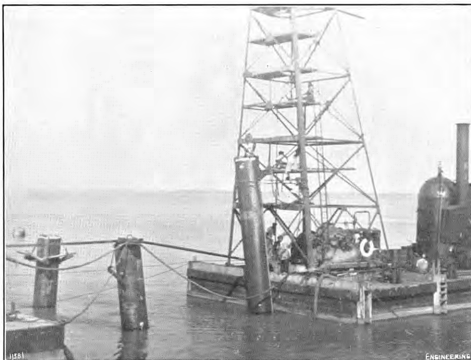
FIG. 14. SINKING PILE WITH WATER JET.
