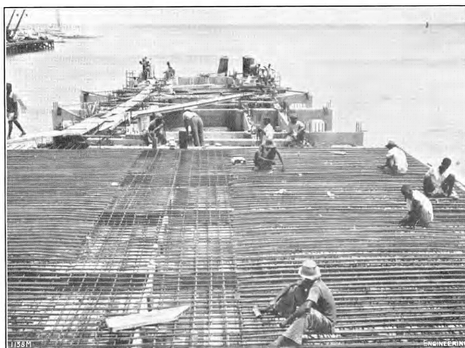
FIG. 17. REINFORCEMENT OF DECK SLAB.
