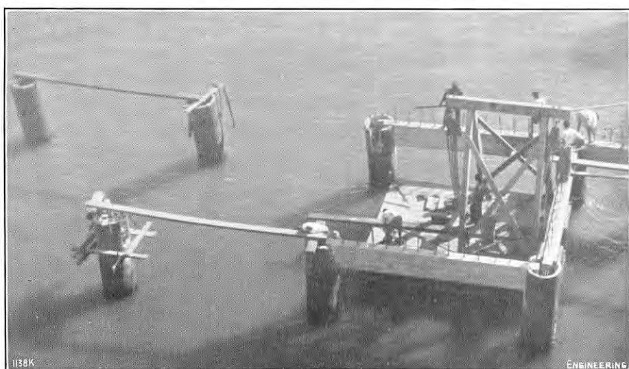
FIG. 15. PLACING PRECAST DECK-BEAMS.
