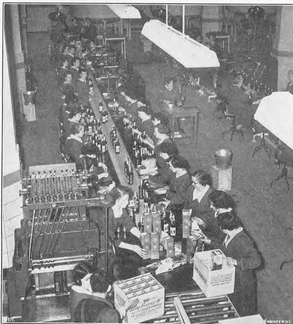
FIG. 1. GENERAL VIEW OF BOTTLING HALL.
