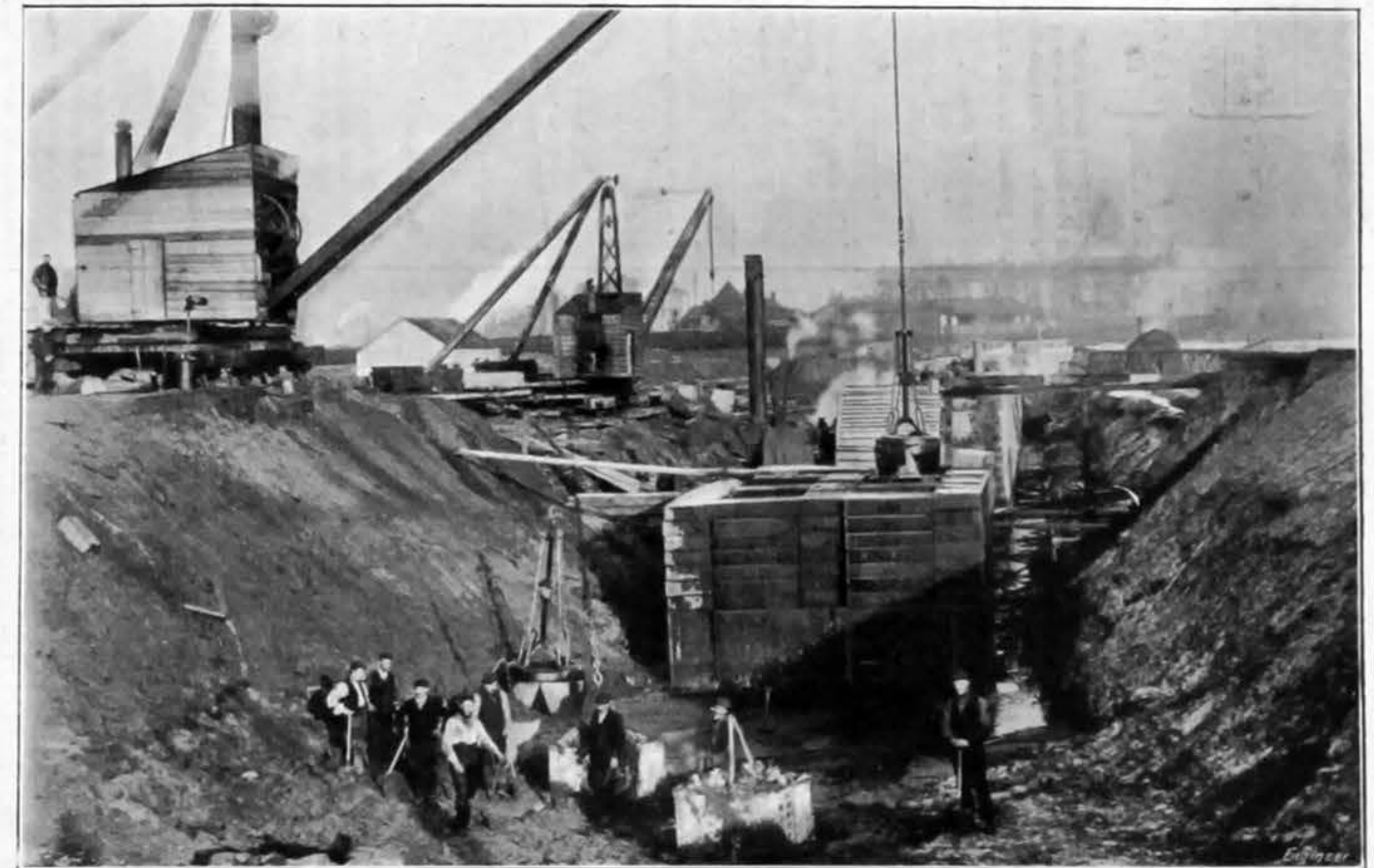
Fig. 4—MONOLITH IN PROCESS OF BEING SUNK
