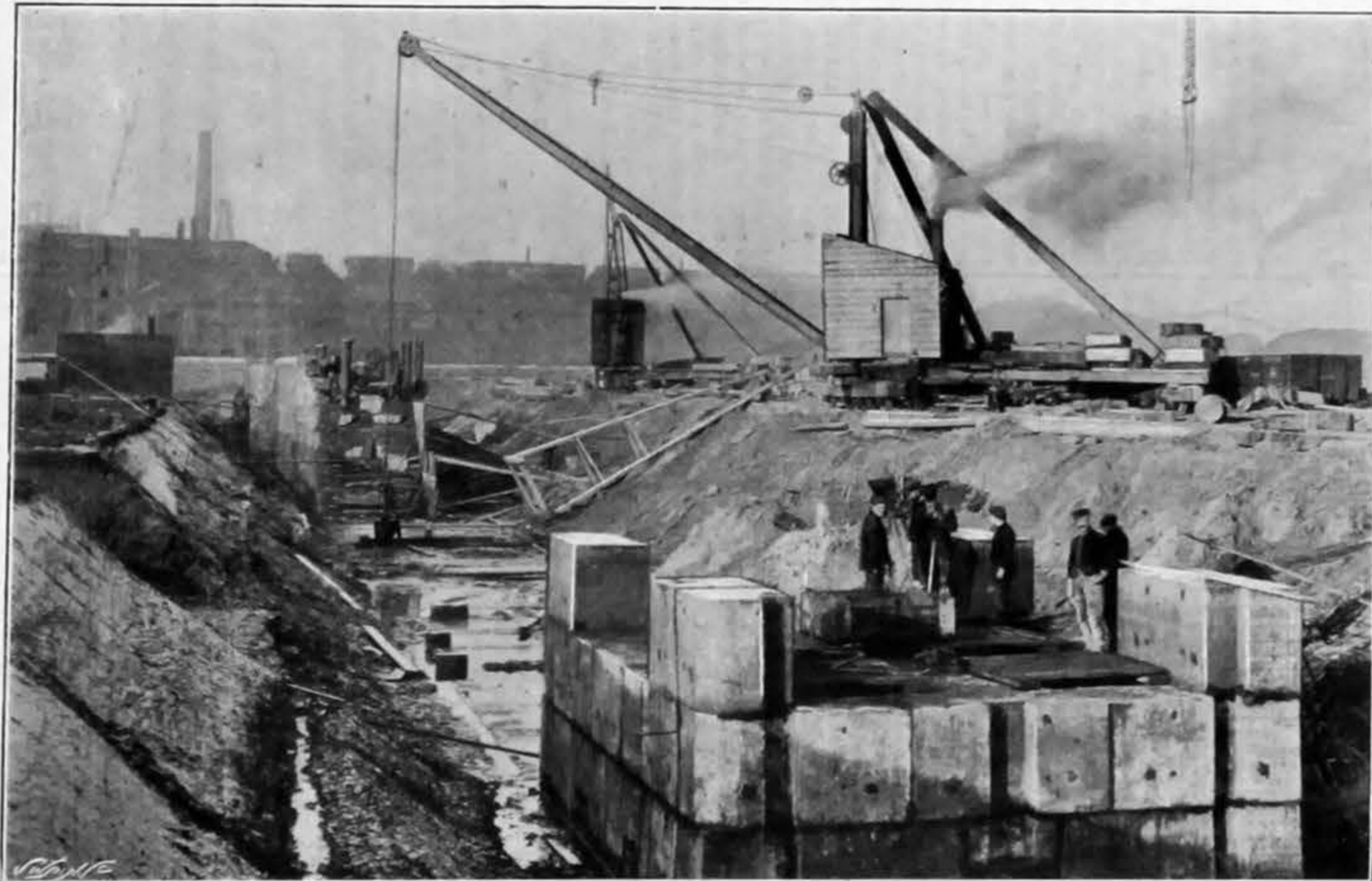
Fig. 3—CONCRETE MONOLITH IN COURSE OF CONSTRUCTION
