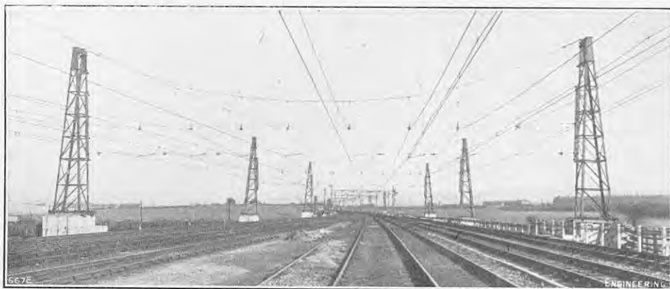
FIG. 5. MULTIPLE-TRACK HEAD-SPAN CONSTRUCTION.
