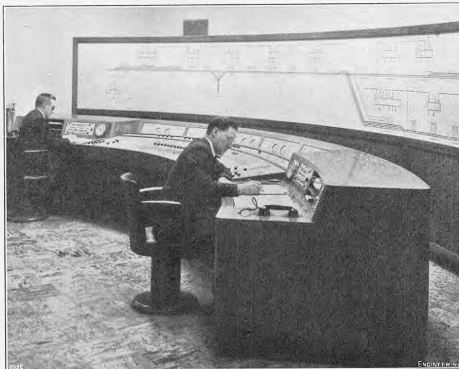
FIG. 5. PENISTONE CONTROL ROOM.
