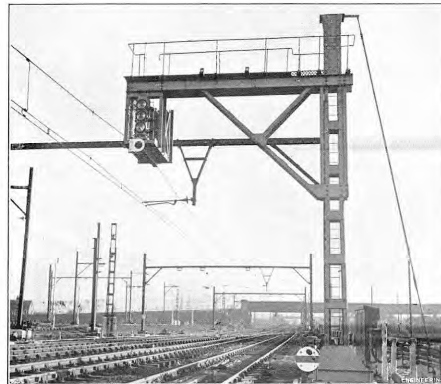
FIG. 11. UP GOODS SIGNAL AT WATH.
