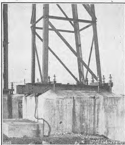
FIG. 6. HEAD-SPAN TOWER BASE.
