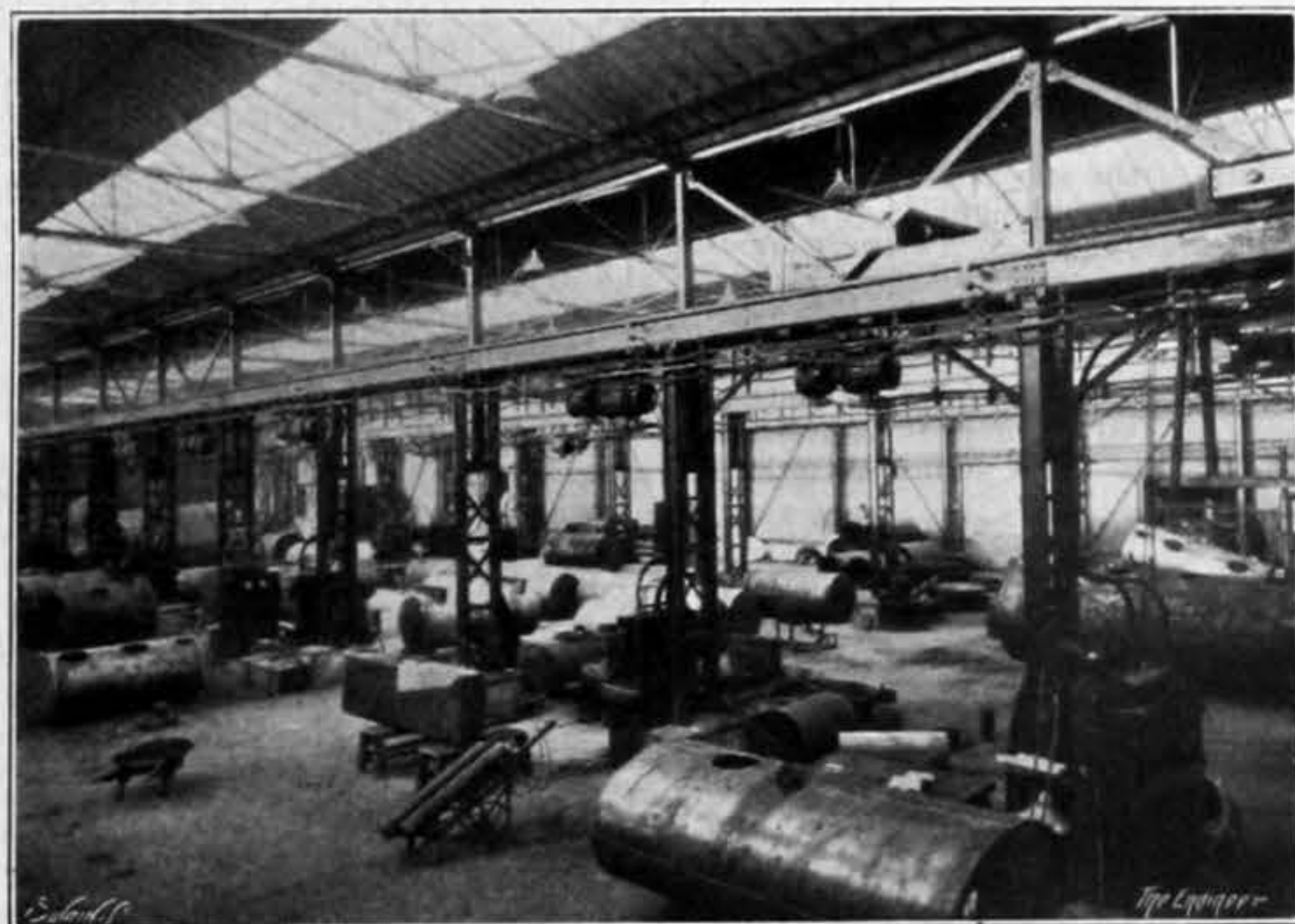
FIG. 2—GENERAL VIEW OF WELDING SHOP
