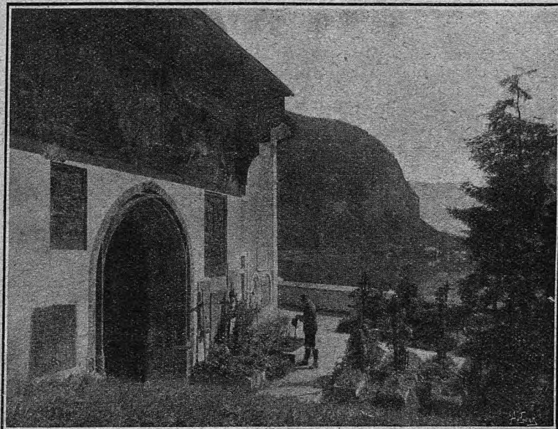
The front of the parish church at Hallsta't, with a view of the Chateau of Groß.
