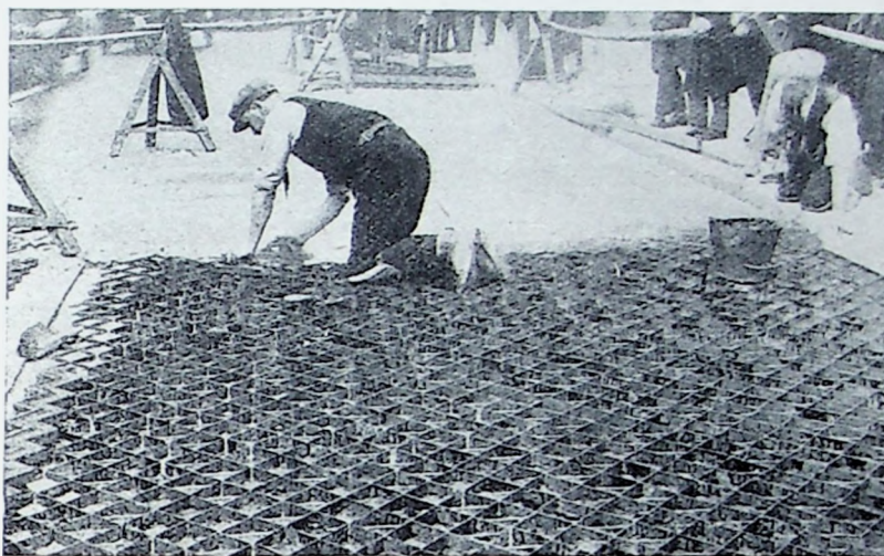
A "Surfasteel" steel-mesh road under construction at Hammersmith Broadway, London. Asphalt is being used as a "filling."
