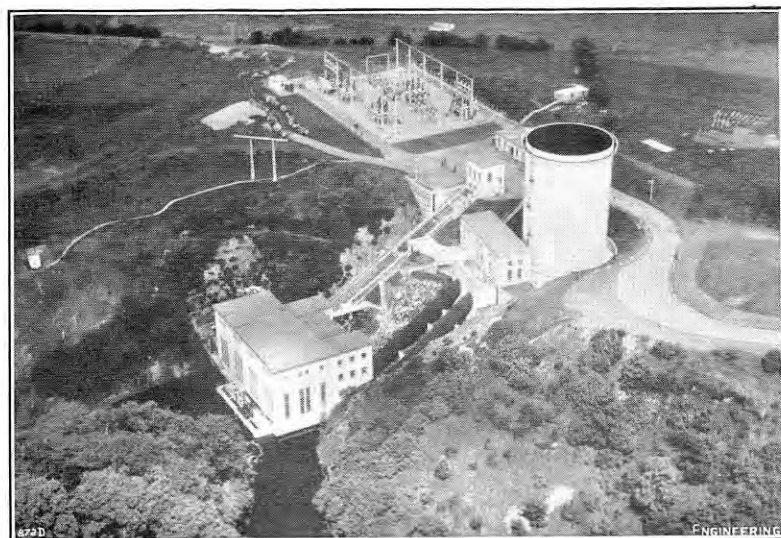
FIG. 4. POULAPHUCA POWER STATION AND SURGE TANK.
