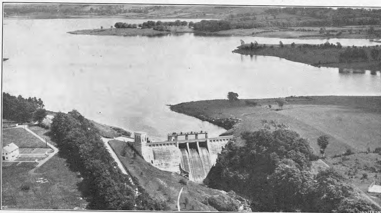
FIG. 1. AERIAL VIEW OF POULAPHUCA DAM.
