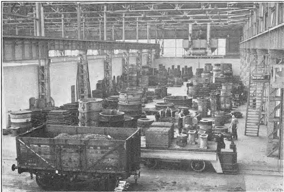
FIG. 5. CHILL STORAGE AREA.
