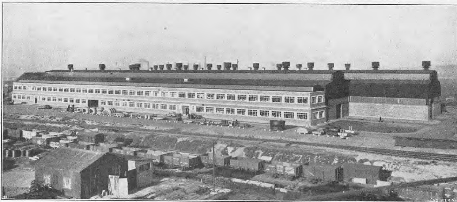
FIG. 1. GENERAL VIEW OF WORKS.
