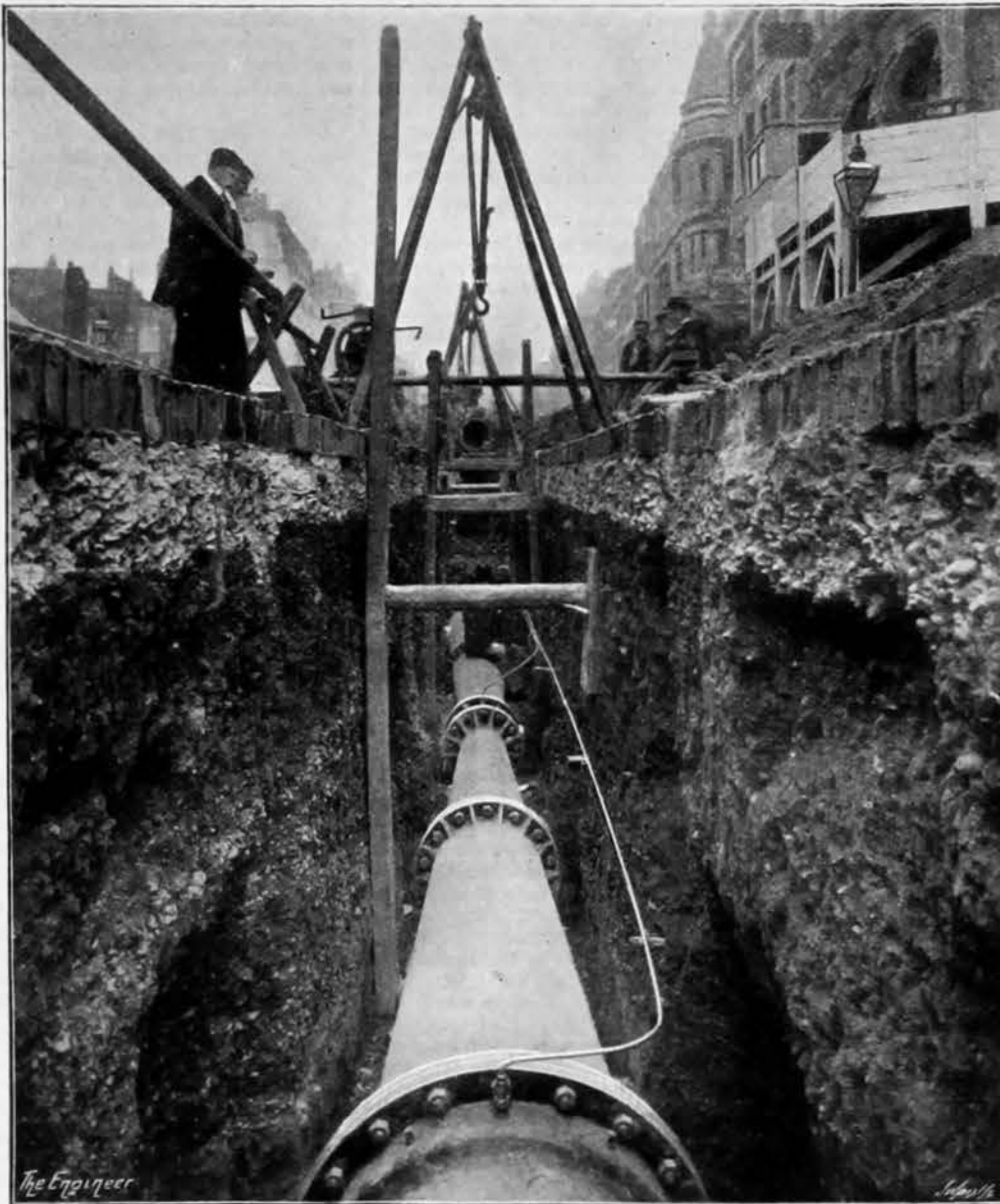
Fig. 2—LAYING TWO-WAY "VENTURI" METER IN LONDON
