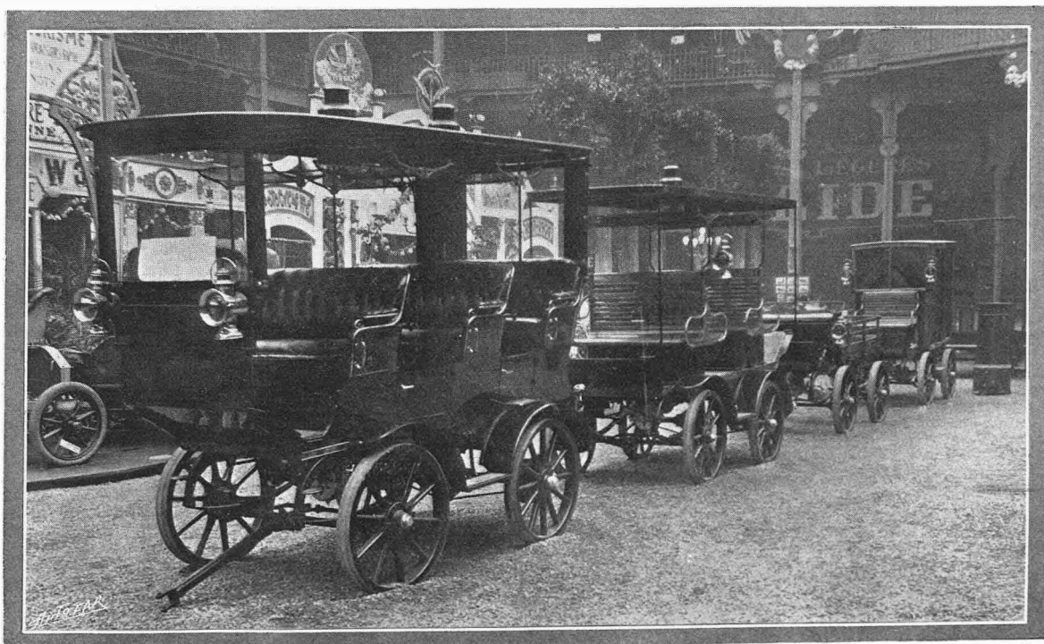
THE RENARD TRAIN. This extraordinary collection of passenger vehicles, which is drawn by a 60 hp. Darracq tractor, excited a great deal of attention. Unfortunately the tractor was not exhibited, but only its train.
