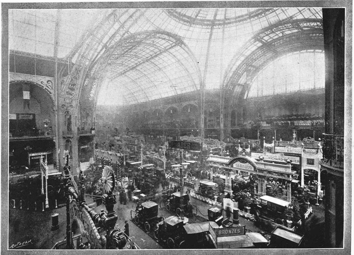
A diagonal view across the Salon from the second gallery in the centre of the building. This view, although an excellent one, only gives a faint idea of the size and general effect of the show. It was taken practically from the centre of the building, but even although only half the length is shown, the perspective as seen by the eye, is considerably more imposing than that rendered by the camera.
