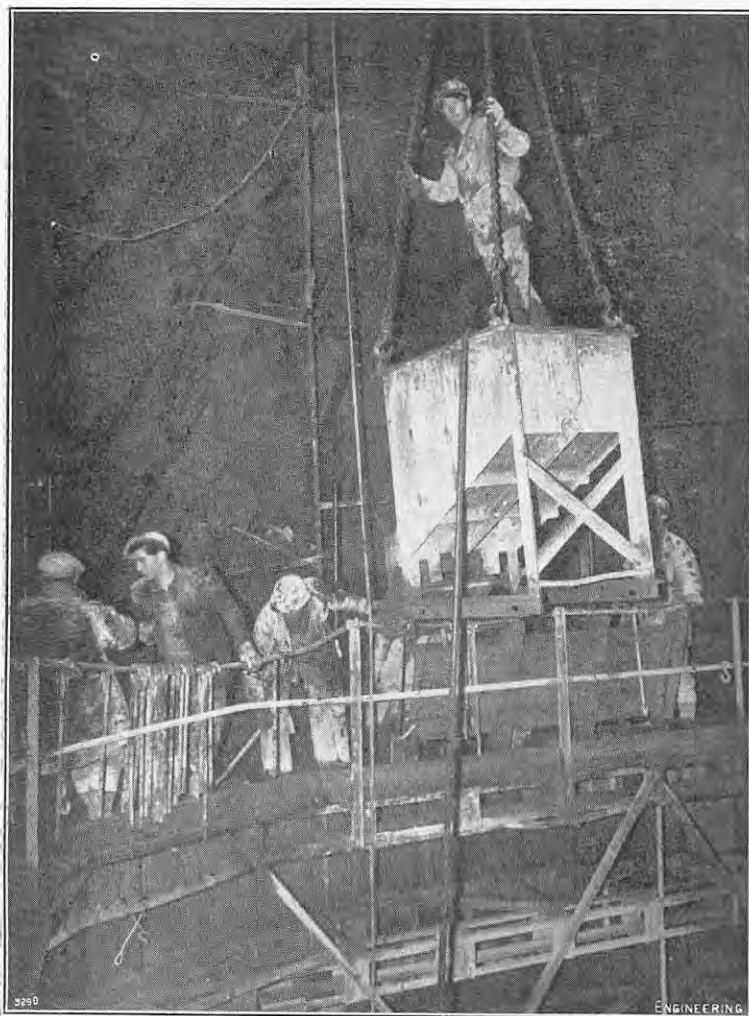
FIG. 19. CONCRETE SKIP AT SHUTTER IN SURGE SHAFT.
