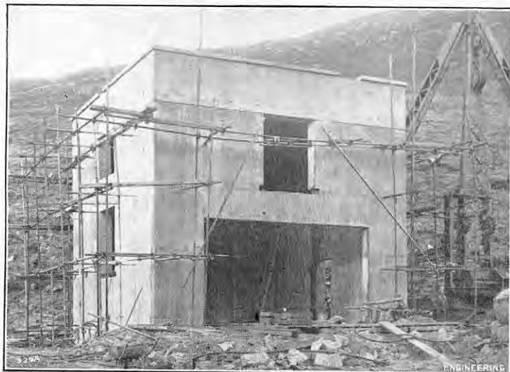
FIG. 1. SCREEN-SHAFT SUPERSTRUCTURE.
