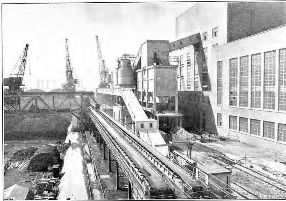
FIG. 2. CONVEYORS AND COAL-HANDLING PLANT.
