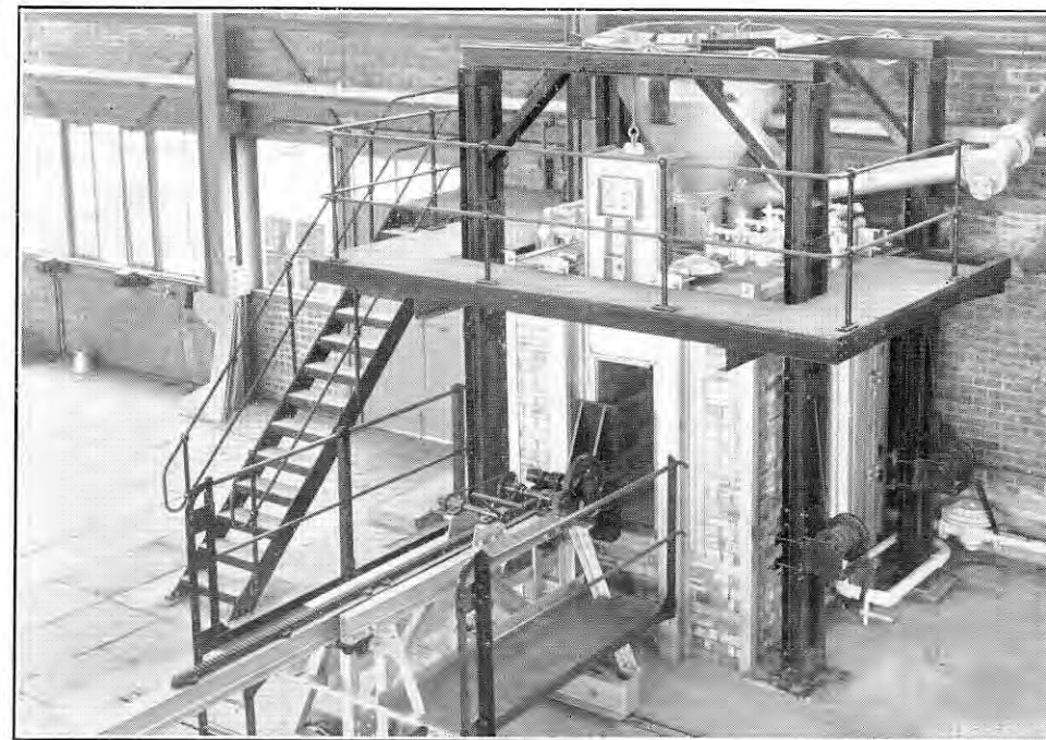
FIG. 4. EXPERIMENTAL COKE OVEN.
