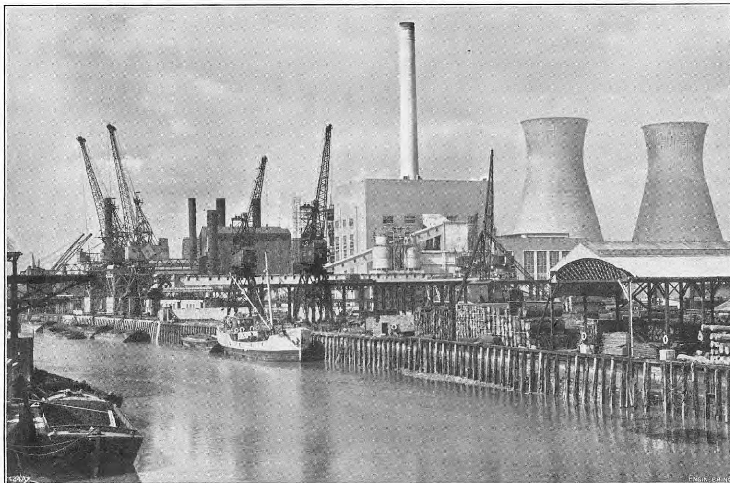
FIG. 1. GENERAL VIEW OF STATION FROM CANNING TOWN BRIDGE.
