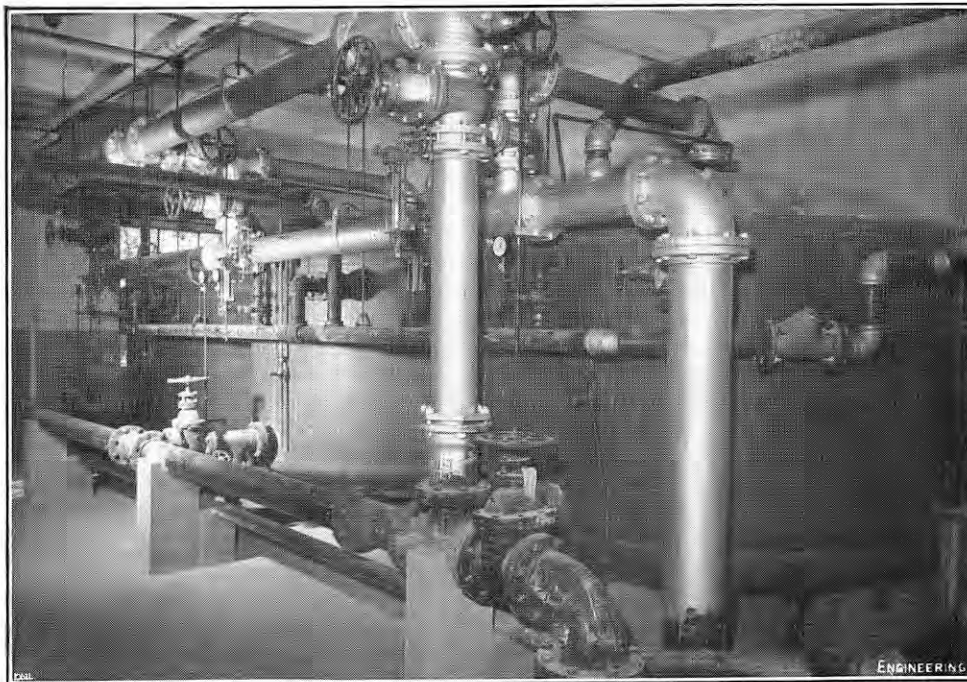
FIG. 13. PRESSURE FILTERS.
