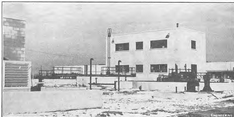
FIG. 1. GENERAL VIEW OF PLANT.
