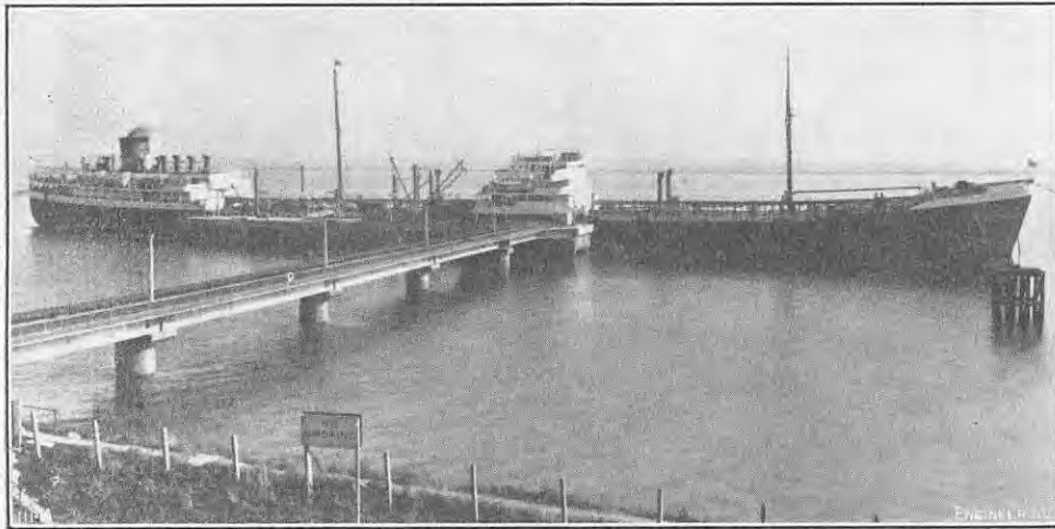
FIG. 1. GENERAL VIEW OF JETTY AND APPROACH.
