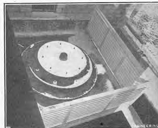
FIG. 16. CASCADE AERATOR.
