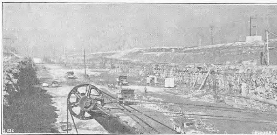
FIG. 4. CONSTRUCTION OF CANAL.
