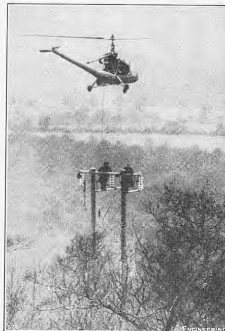
FIG. 2. SECURING CORD TO POLE CROSS-ARM.
