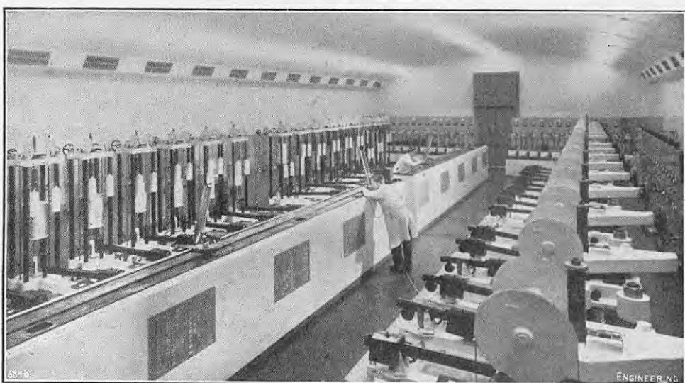
FIG. 2. MAIN TESTING LABORATORY.
