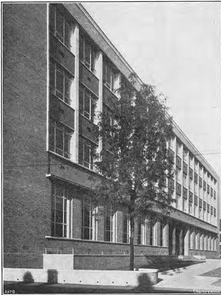
FIG. 2. FRONTAGE OF STEPHENSON BUILDING.
