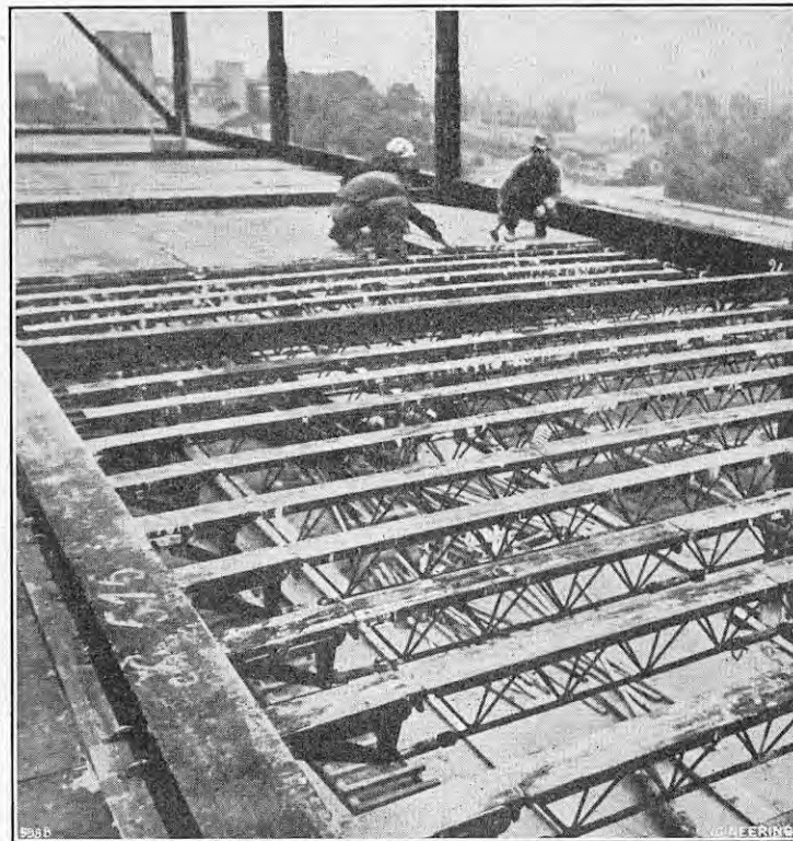
FIG. 2. TYPICAL LAYOUT OF CENTRING.
