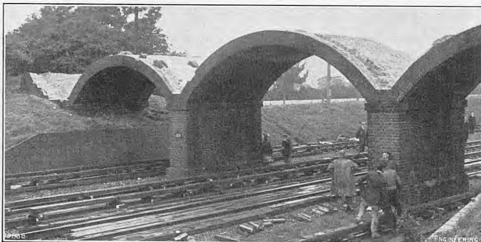
FIG. 1. BRIDGE PREPARED FOR DEMOLITION.
