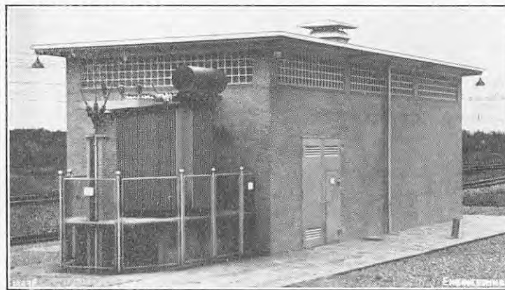
FIG. 6. EXTERIOR OF FIXED SUBSTATION.
