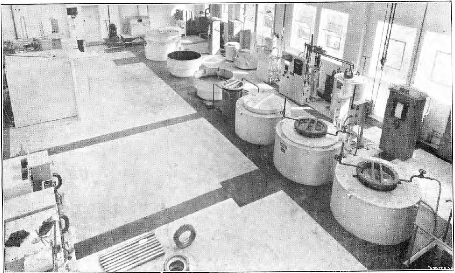
FIG. 3. GENERAL VIEW OF HEAT-TREATMENT SHOP AND EQUIPMENT.
