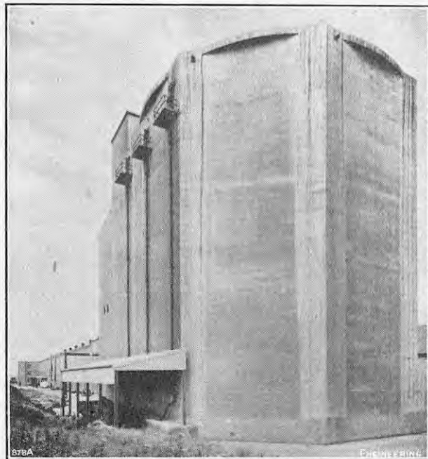
FIG. 1. MIXING TOWER WITH SUCTION PIPES.
