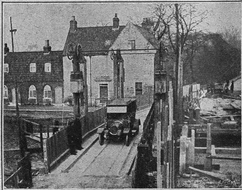
A TEMPORARY WOODEN DRAWBRIDGE. The old bridge which spanned the river Hull near Beverley, Yorkshire, was a notorious danger spot, but a contract has been placed for an iron swing bridge operated by hydraulic power. The old stone structure has been removed and a temporary wooden drawbridge across the river has been installed alongside the site of the new one, and a man is stationed with red and green flags to signal if the road be clear or not to approaching traffic. The new bridge is expected to be finished about the end of July this year, and will be of great benefit to road users going into Holderness from the west, as there is no bridge for ten miles on either side of this spot, which lies about 1½ miles due east of Beverley, on the Hornsea road.
