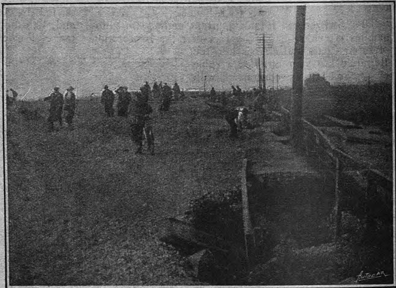
For a considerable distance between Lancing and Worthing the sea during the great Easter storm covered the Brighton-Worthing road with thousands of tons of shingle, in some places to a depth of three or four feet, and some great holes like that shown on the right of the picture were scored in the roadway.
