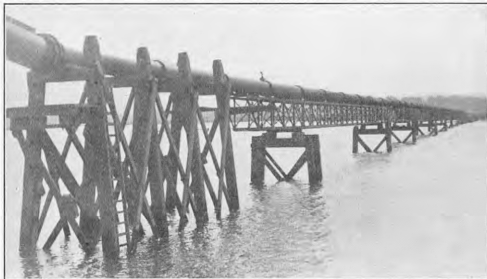
FIG. 4. PIPELINE JETTY FROM DREDGER TO RECLAMATION AREA.
