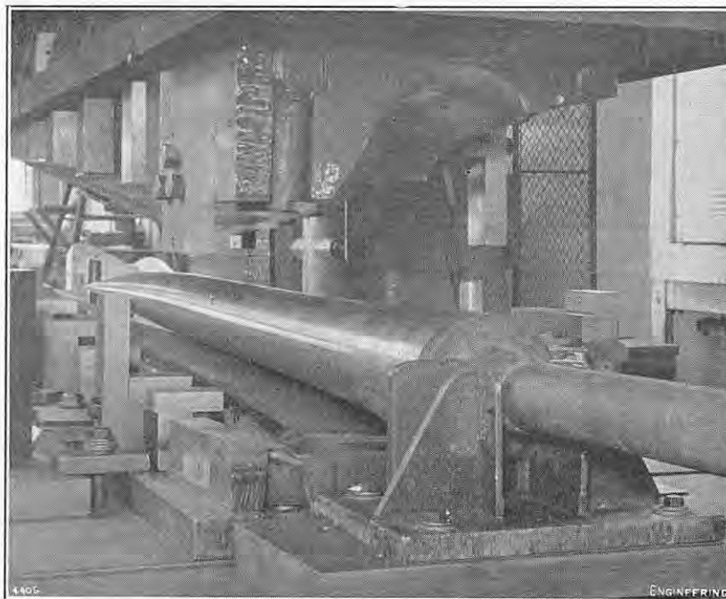
FIG. 8. CORE TUBE LOCATED IN DIES OF HOT-FORMING PRESS.
