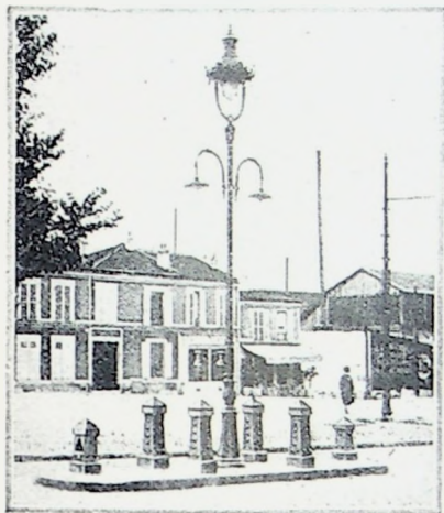
The new illuminated refuges now being tried out in Paris consist of a number of concrete pillars in which are red reflectors.
