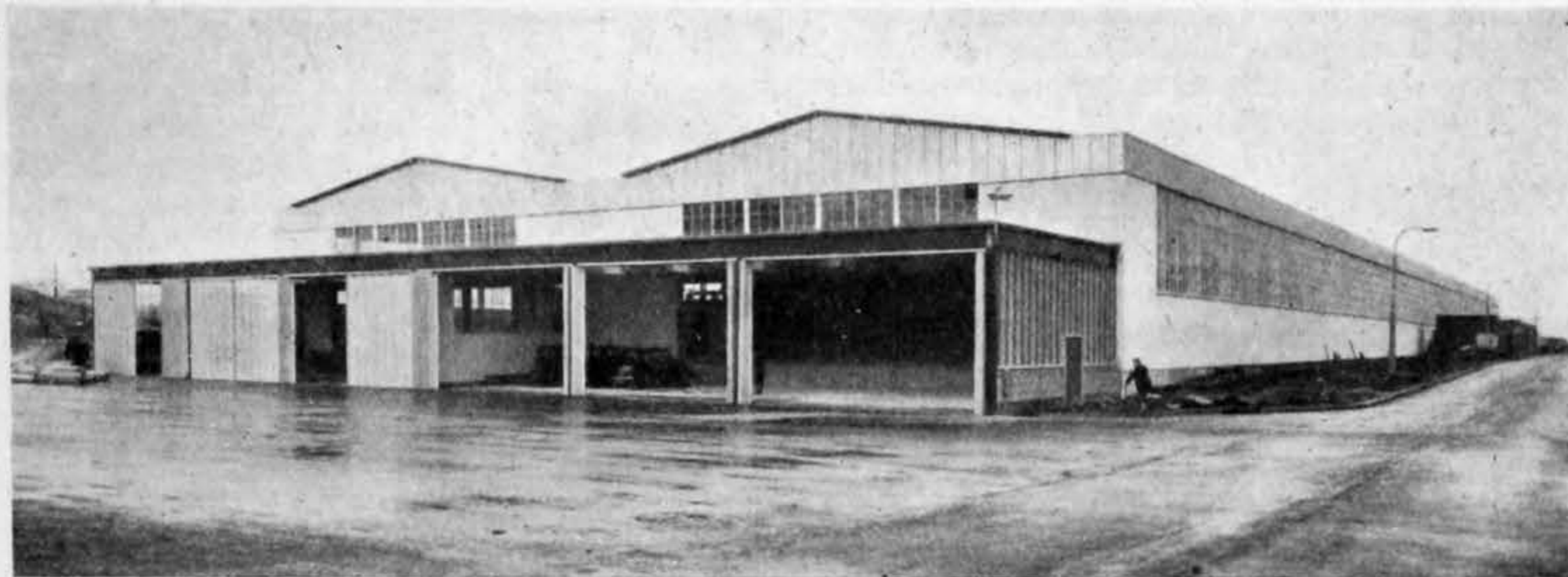
Exterior view of factory looking from the off loading end
