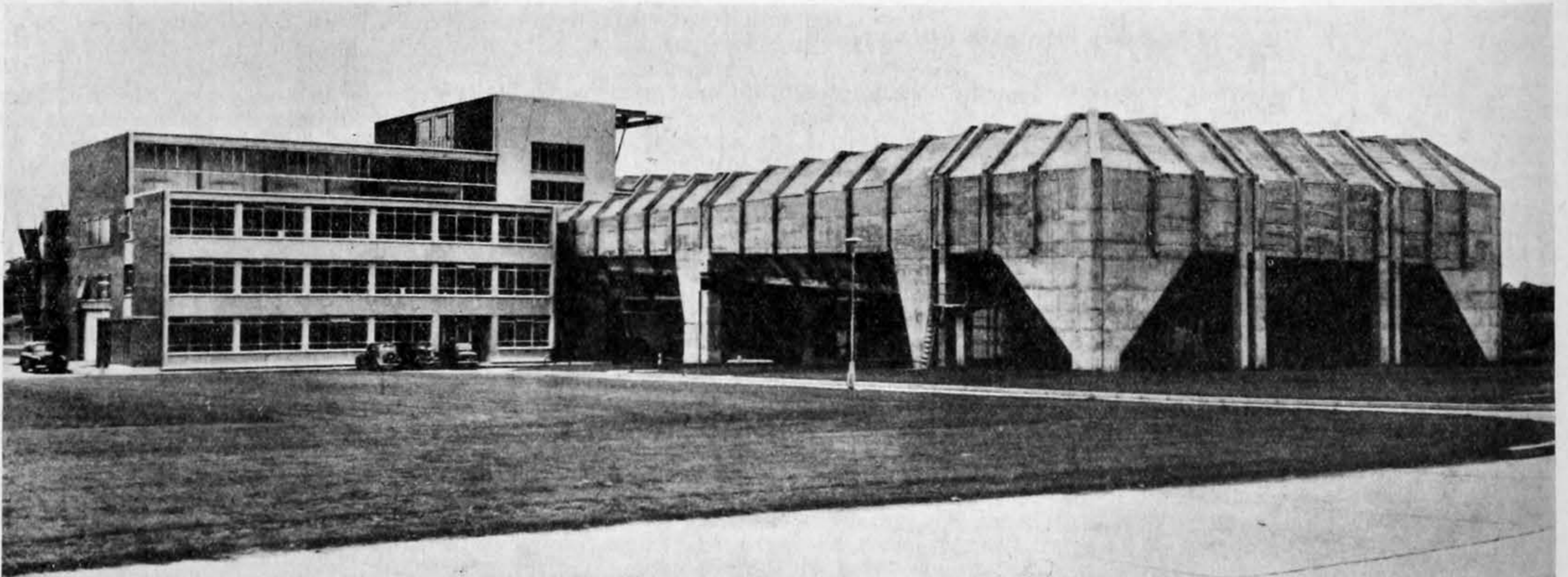
13ft by 9ft reinforced concrete low-speed wind tunnel at Bedford
