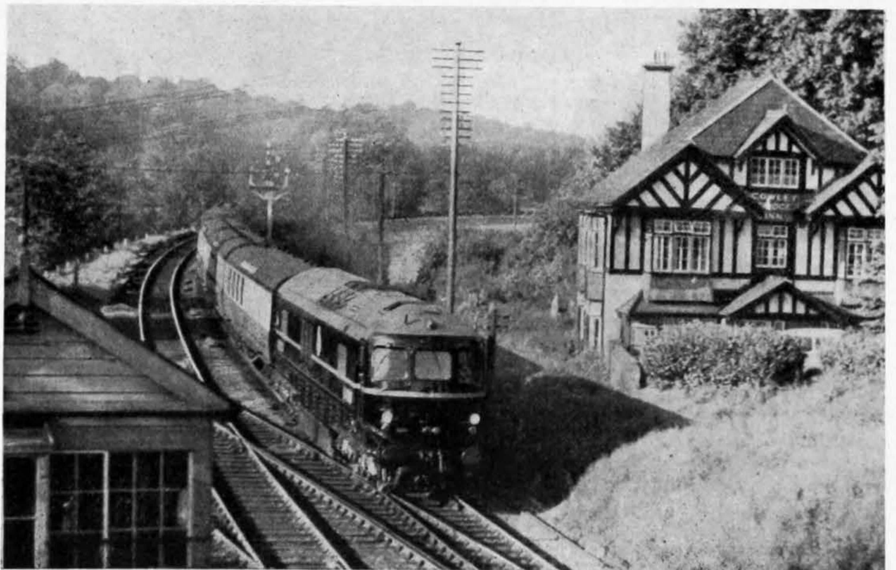
Western Region, gas turbine engine on Penzance express
