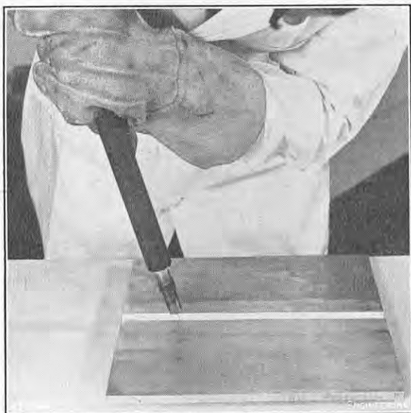
FIG. 1. WELDING GUN IN USE.
