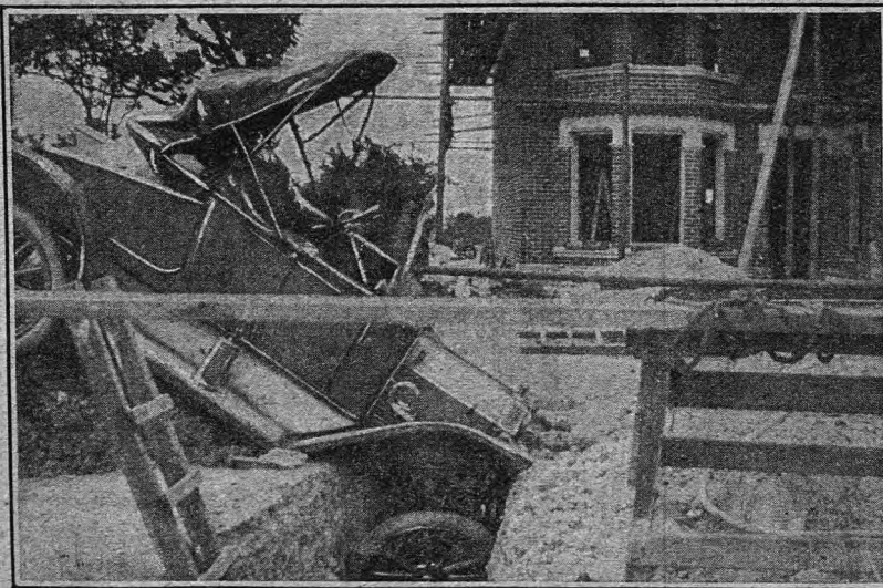
A car in a 10 ft. trench. Whilst driving recently at 11 p.m. between Weymouth and Dorchester, a doctor failed to understand the arrangement of the lights round a trench, cut partly across the road, and charged a 4 ft. bank of earth, surmounted it and dropped into the trench as shown above. The doctor was, fortunately, not seriously hurt.
