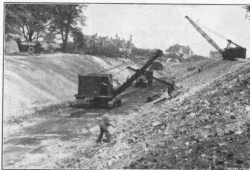
FIG. 3. USING DRAG LINE EXCAVATOR AND FACE SHOVEL.
