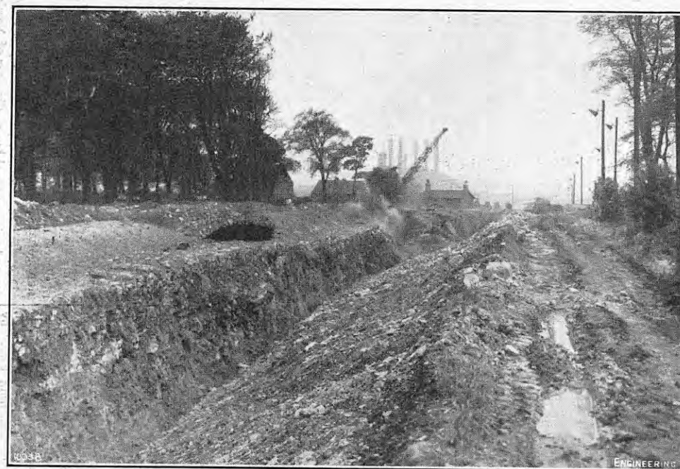
FIG. 2. DEMOLITION BY EXPLOSIVES.
