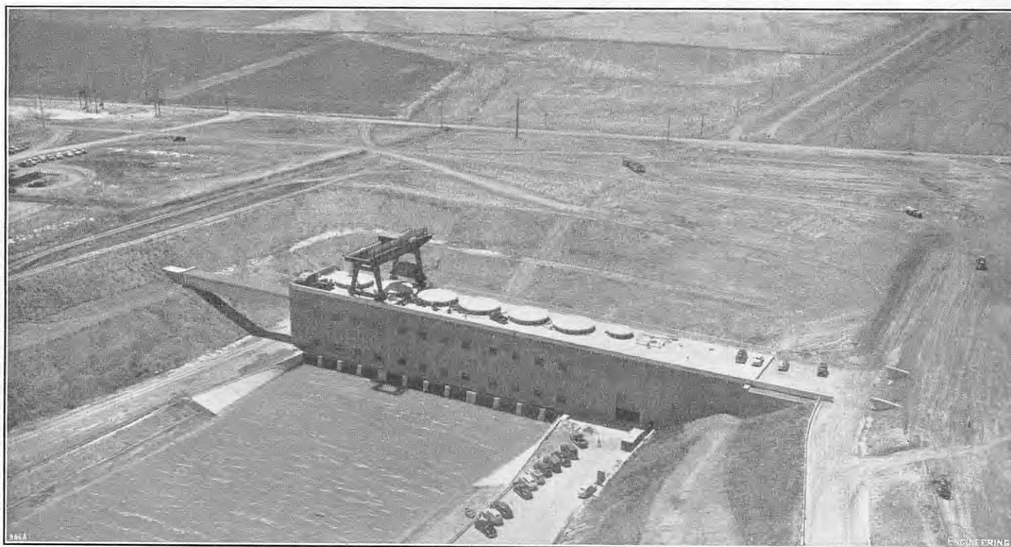
FIG. 1. AERIAL VIEW OF PUMPING STATION.
