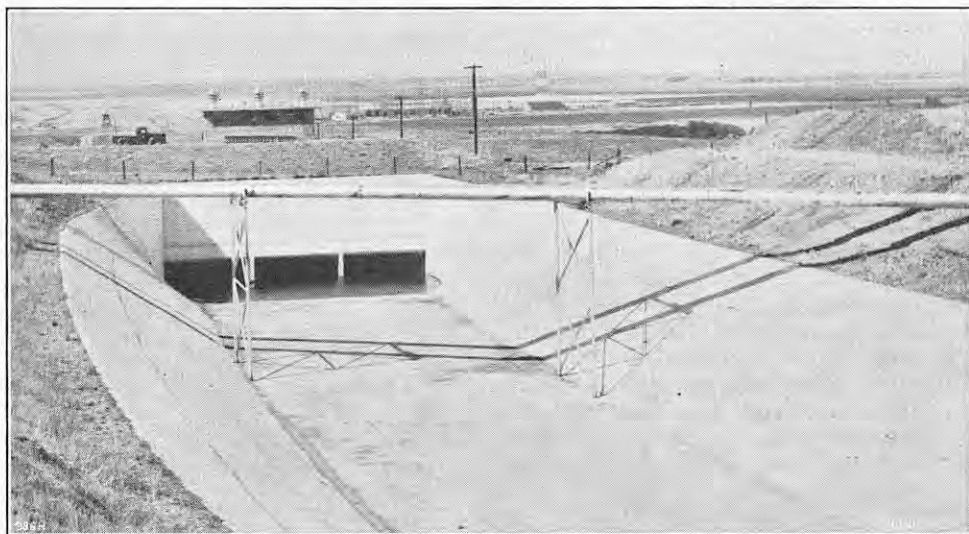
FIG. 4. OUTLET STRUCTURE FOR DISCHARGE PIPES.
