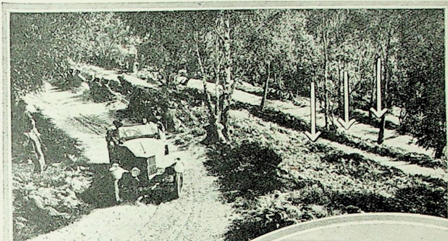
THE CORKSCREW. Known affectionately — or otherwise — as "the Corkscrew," Inverfarigaig rises in a series of terraces each approached by an acute hair-pin bend. The photograph shows four of these terraces, three in the background being identified with arrows. Many cars are forced to reverse in order to negotiate the difficult turns.
