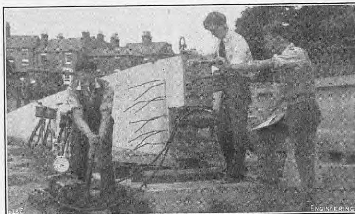
FIG. 5. POST-TENSIONING OPERATION ON PRE-CAST BEAMS.
