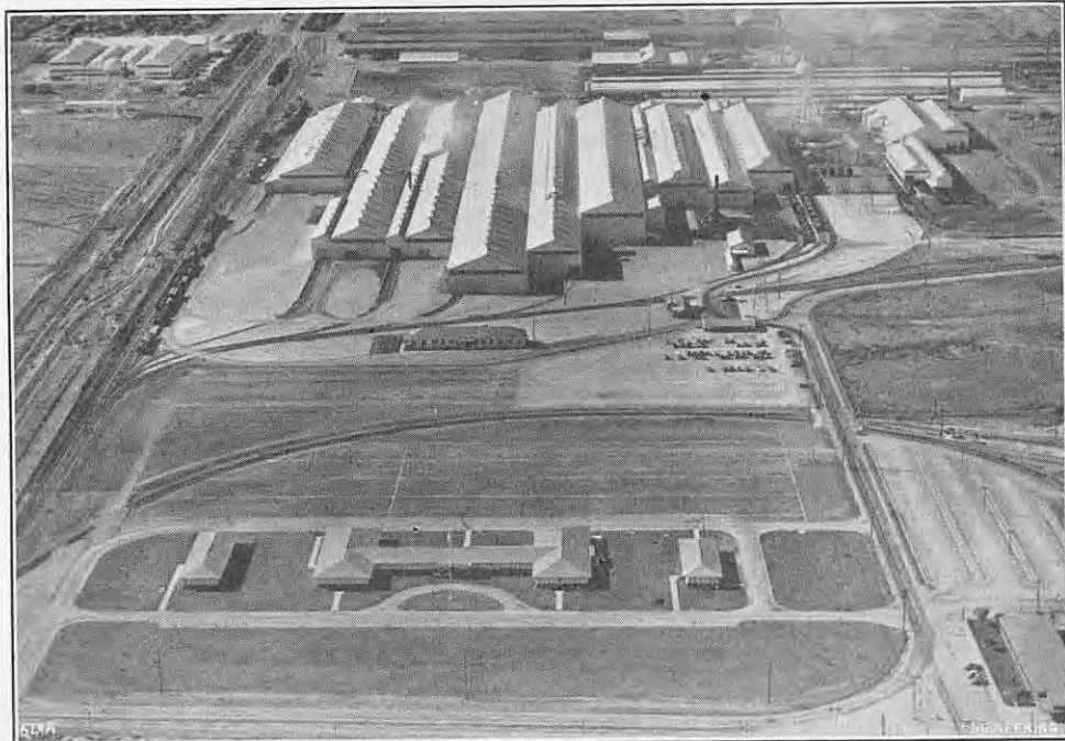
FIG. 1. GENERAL VIEW OF PLANT.
