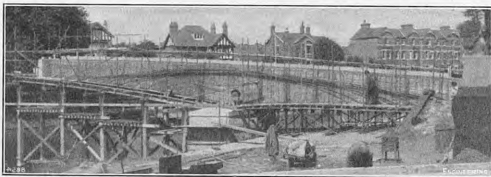
FIG. 2. CENTRE CANTILEVER ON SOUTH SIDE, UNDER CONSTRUCTION.
