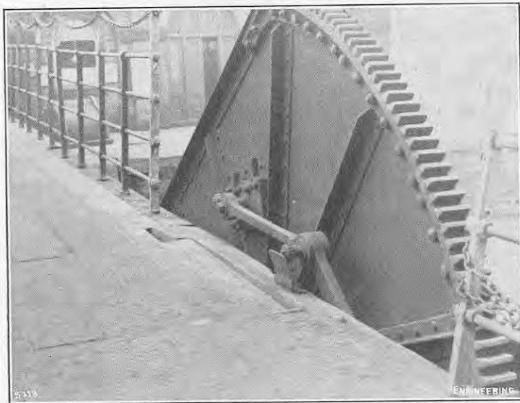
FIG. 2. LINK MECHANISM.
