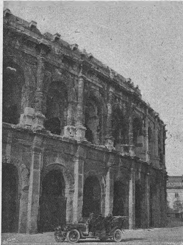
Fig. 3.—The Roman amphitheatre at Nîmes, where bull fights are still held in the summer months. The whole building is composed of great cubes of stone perfectly mortised without mortar.
