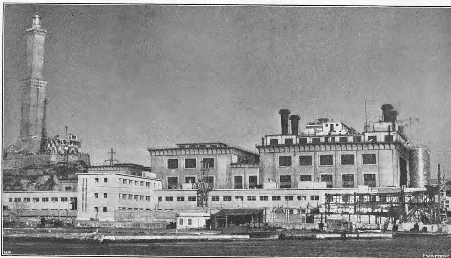
FIG. 1. THE "CONCENTER" POWER STATION, GENOA.
