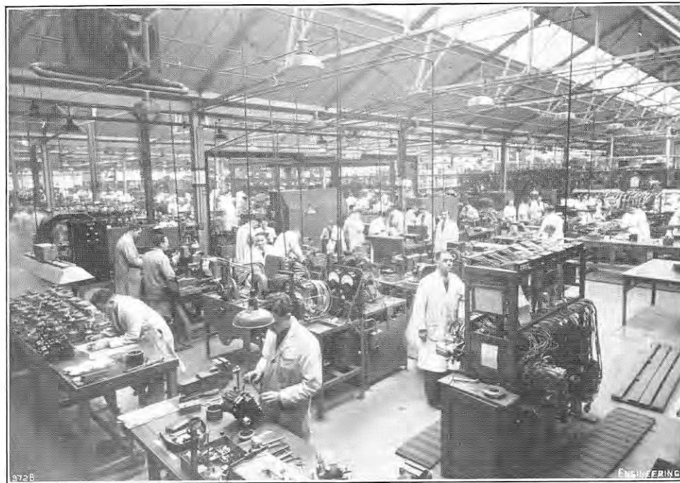
FIG. 9 MAGNETO AND HARNESS OVERHAUL BAY.
